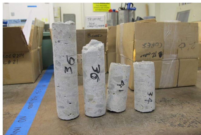
Image 1: Bridge cores; cores equal to or longer than 3 inches were used for ASR visual inspection
