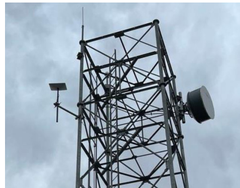
Image 1: Starlink high-performance antenna (left side of image) after installation at the Redding Fiber Hub – Image Source - AHMCT
