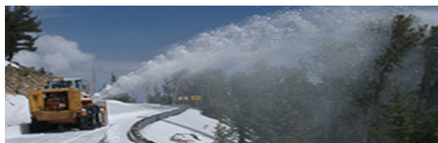
Image 1: Rotary blower removing snow from roadway
