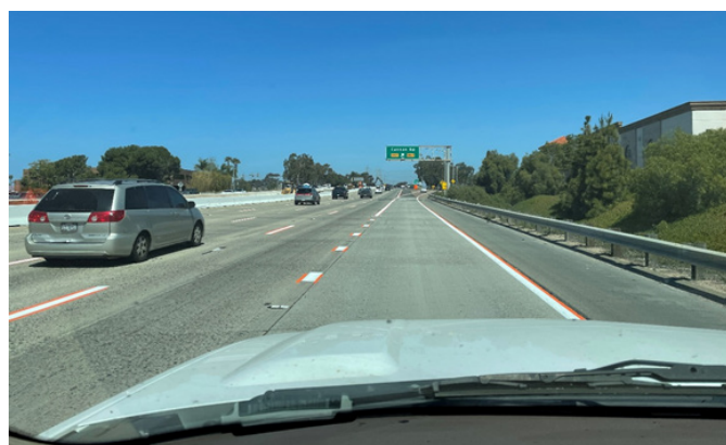
Image 3: Caltrans District 11 temporary work zone pavement delineation pattern – alternative 2
