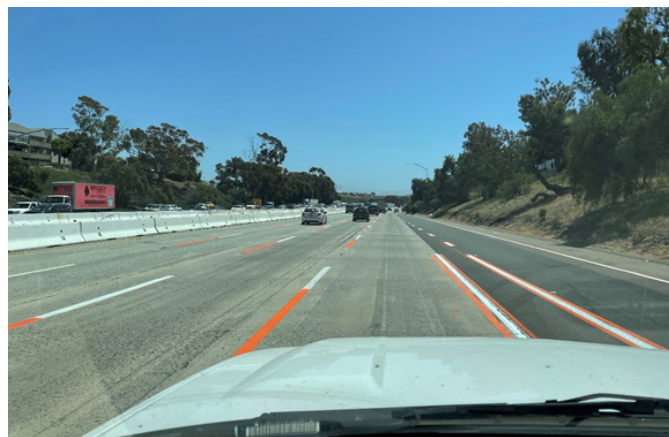
Image 2: Caltrans District 11 temporary work zone pavement delineation pattern – alternative 1
