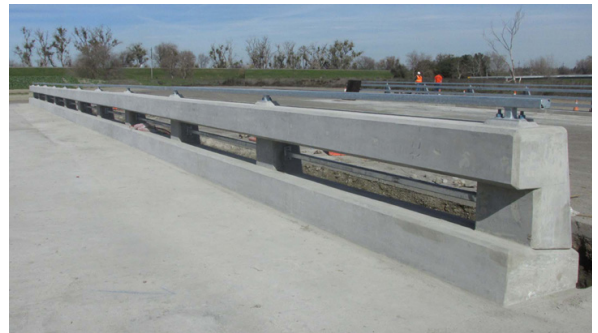
Image 2: Completed Type 85 Bridge Rail at the Caltrans Dynamic Test Facility
