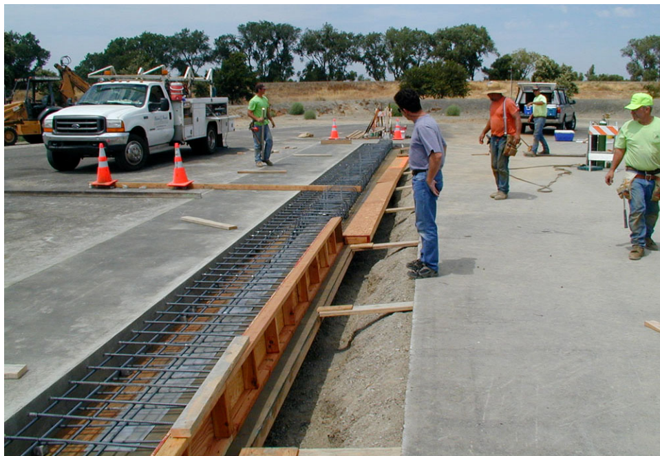
Figure 2-5 - Overhang Steel and Forms
