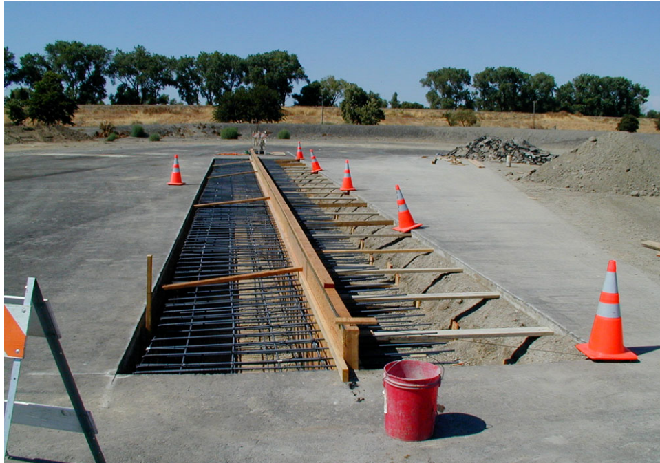
Figure 2-4 - Anchor Block Reinforcing Steel and Forms
