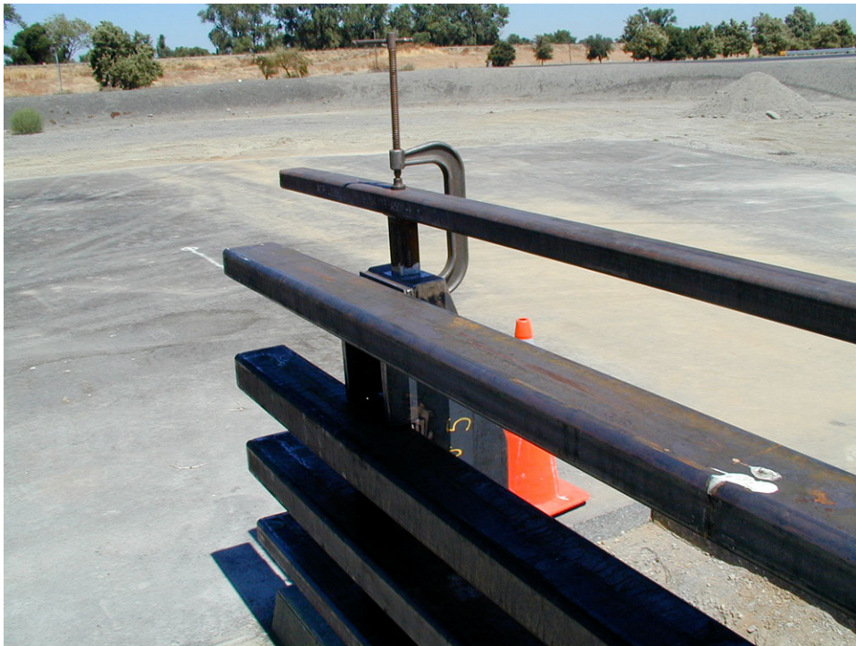
Figure 2-8 - Handrail Position and Weld Set-up
