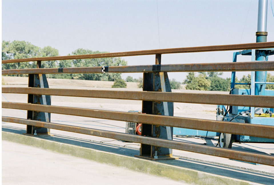
Figure 2-9 - Completed ST-20 Barrier Prior to Testing
