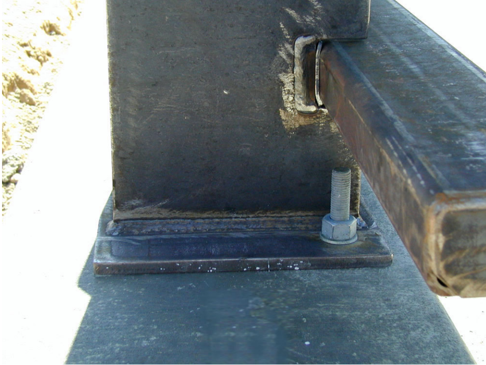
Figure 2-7 - Post-to-Curb Connection
