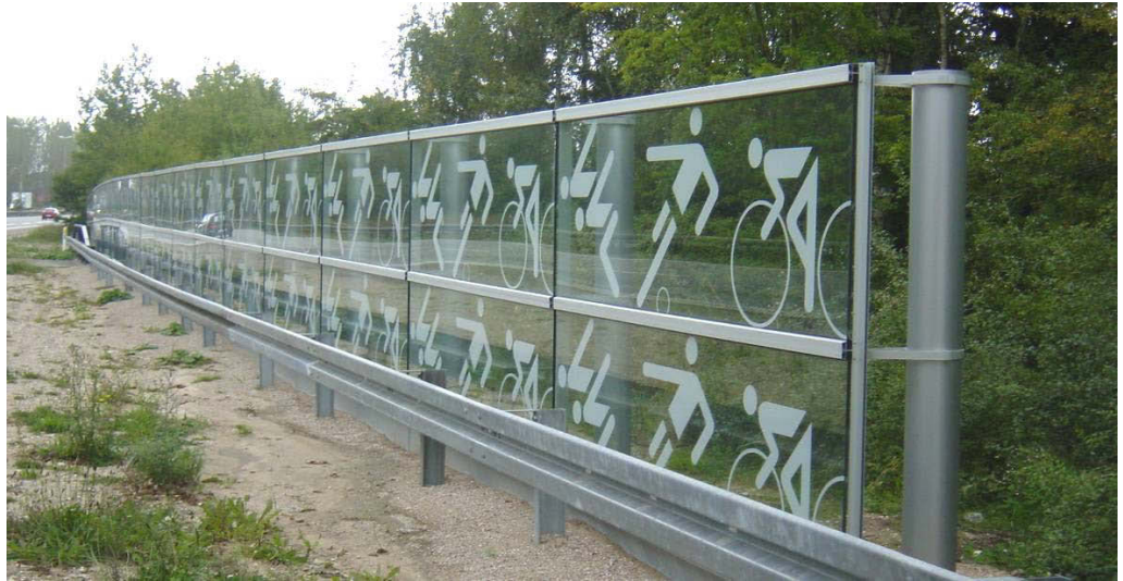
Figure 3.27. Transparent noise barrier with a "bike print" along a highway in an urban district in Denmark [2].
