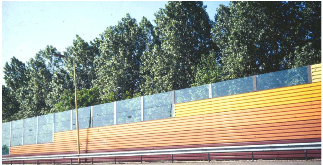
Figure 3.10. 4.5 m (15 ft) high noise barrier with light yellow color at the top and dark red colors below. There is a transparent part and high vegetation behind this barrier at Highway A9 in the Netherlands [3].
