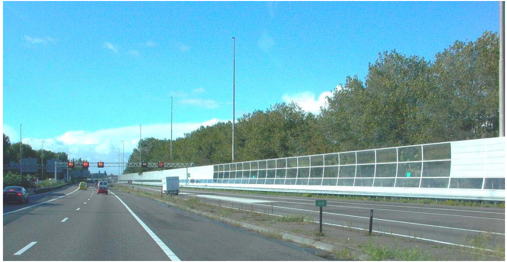
Figure 3.29. Dutch curved steel noise barrier with long transparent section.
