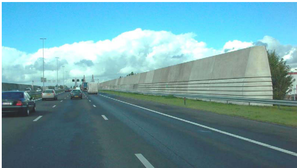
Figure 2.10. Dutch concrete noise barrier bent at a small angle from the road in order to reflect the noise upwards to reduce the disturbance of residents on the other side of the highway.
