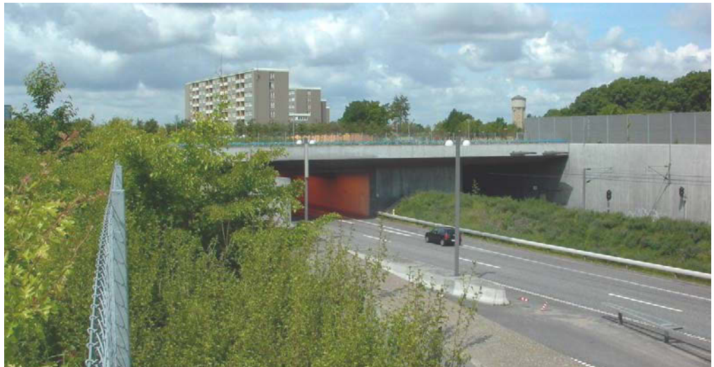
Figure 2.1. 700m long concrete cover over a new highway alignment to Copenhagen Airport through a preexisting residential area with apartments. The cut-and-cover strategy used here solved two problems; reducing traffic noise levels and keeping the new roadway from dividing the community. The covering has been planted and established as a green recreational area.
