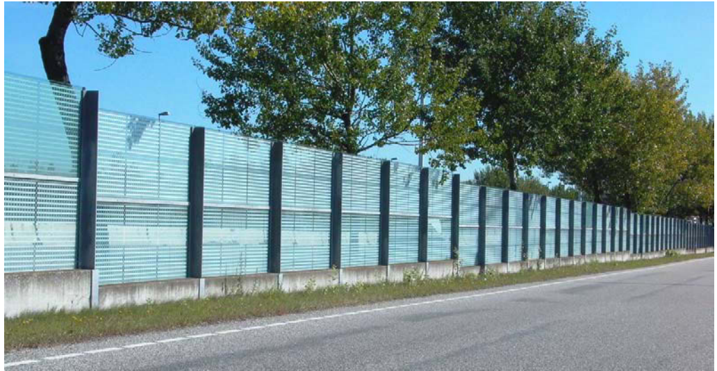
Figure 2.8. 2½ m high transparent noise barrier reflecting noise to the other side of the road along Highway M14 north in Gentofte of Copenhagen, Denmark [1].
