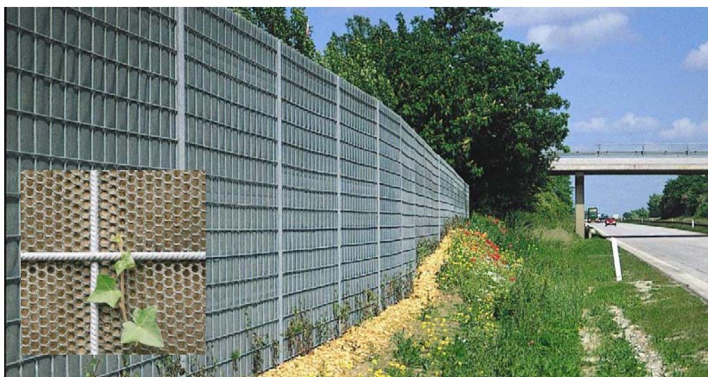
Figure 2.12. Danish absorbing noise barrier made as a steel frame with absorbing mineral wool and a steel grid in front (close up in left corner).
