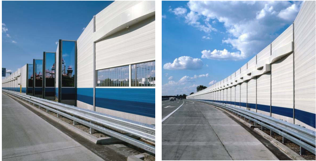
Figure 3.31. Steel and transparent noise barrier along highway in Vienna, Austria.
