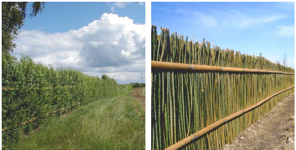
Figure 3.36. Green noise barrier made of panels with willow branches at both sides. When newly constructed to the right and after getting green to the left [2].
