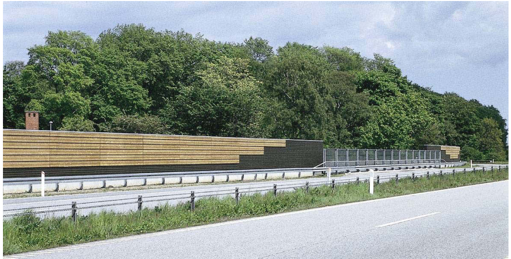
Figure 3.11. Transparent section as part of long wooden noise barrier where Highway M30 passes over a local road in Saksøbing in Denmark [1].
