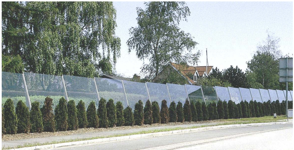
Figure 2.9. 2 m high Transparent noise barrier tilted away from the road in order to reflect the noise upwards to reduce the disturbance of residents on the other side of the road, at National Road 152 in Næstved, Denmark [1].
