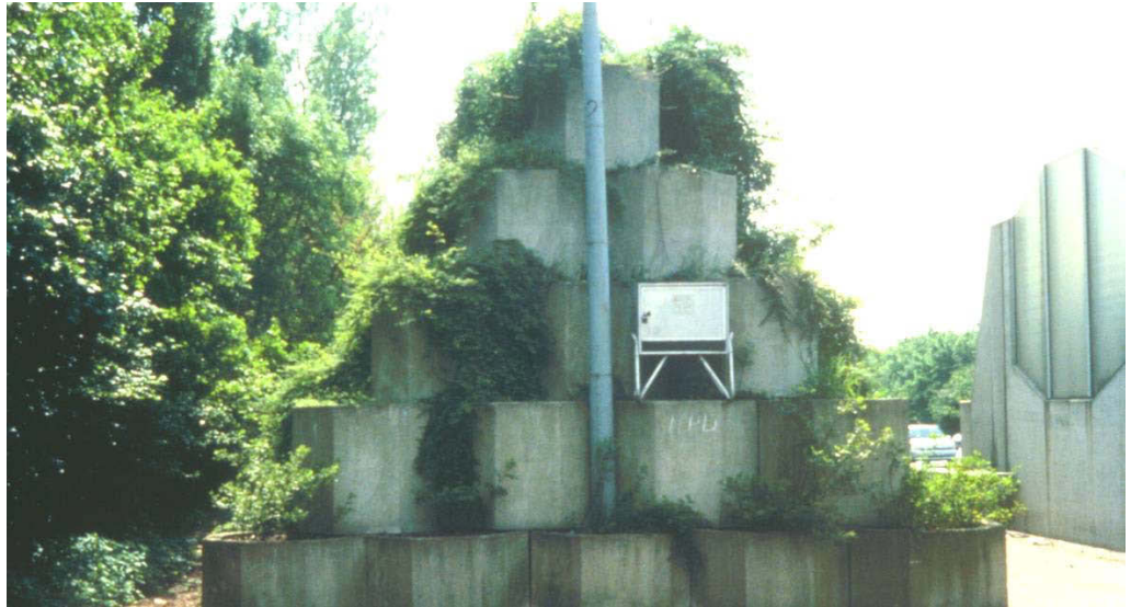
Figure 3.22. Supported earth embankment made of concrete pipes piled on top of each other in triangles and filled with earth along Highway A3 near Cologne in Germany [3].
