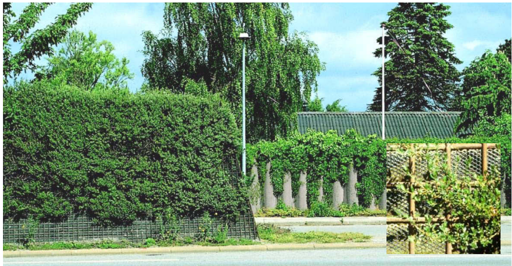
Figure 3.21. A supported 3 m (10 ft) high earth embankment with a slanting steel net to the left (details to the right) at National Road 405 in Aarhus, Denmark [3].
