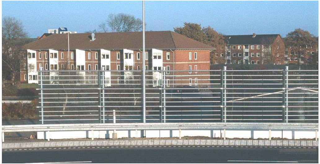
Figure 3.9. Transparent noise barrier along Danish highway in an urban area [2].
