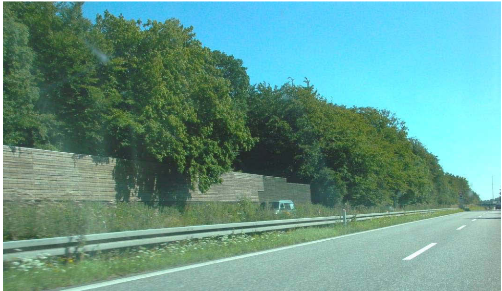
Figure 1.4. Brown wooden noise barrier adapted to the green surroundings on Highway M11 west of Roskilde, Denmark.
