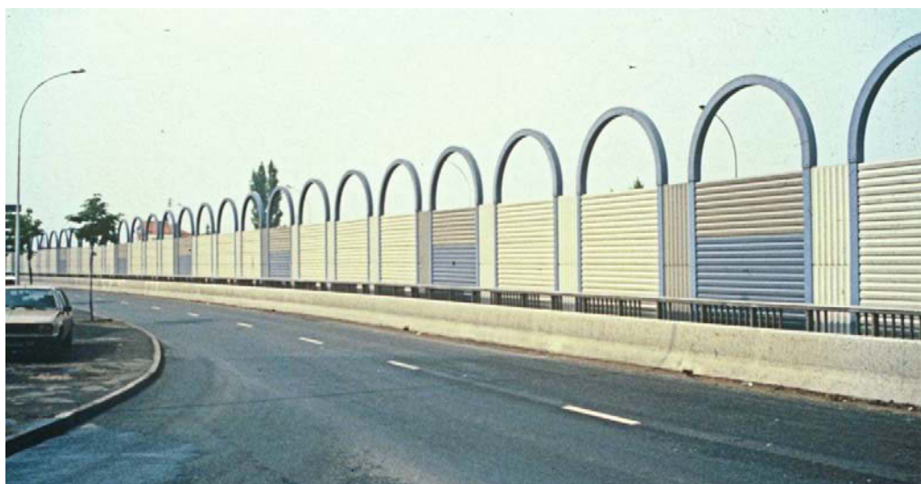
Figure 2.18. 4 m high noise absorbing steel barrier with perforated surface and absorbing material at Highway A6B in Paris, France [3].
