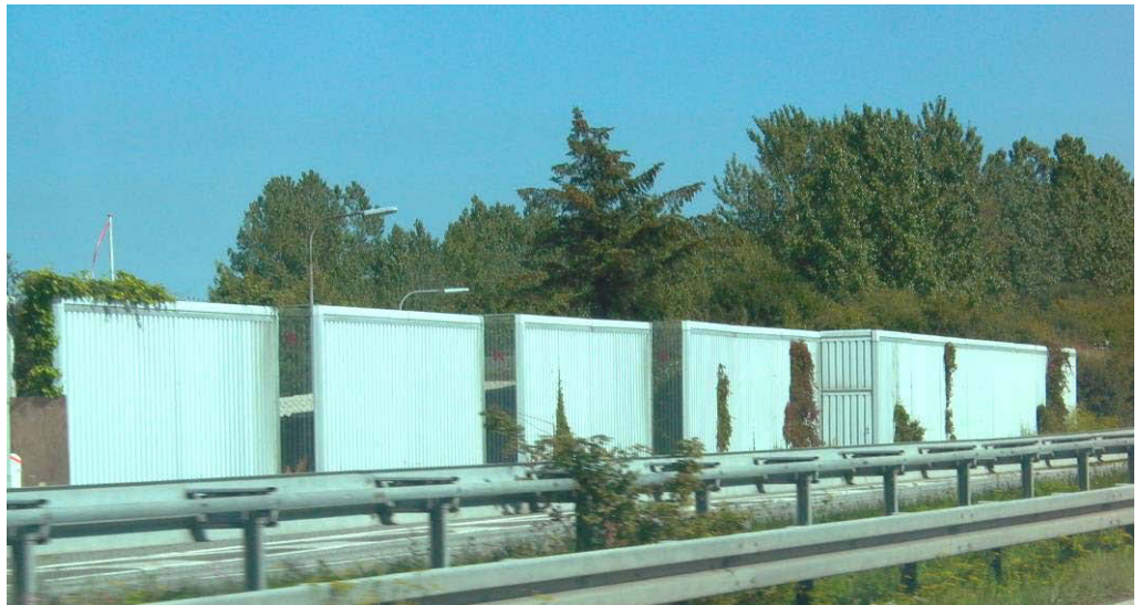
Figure 3.30. PVC barrier with vertical transparent elements along Highway M40 at Nyborg, Denmark.
