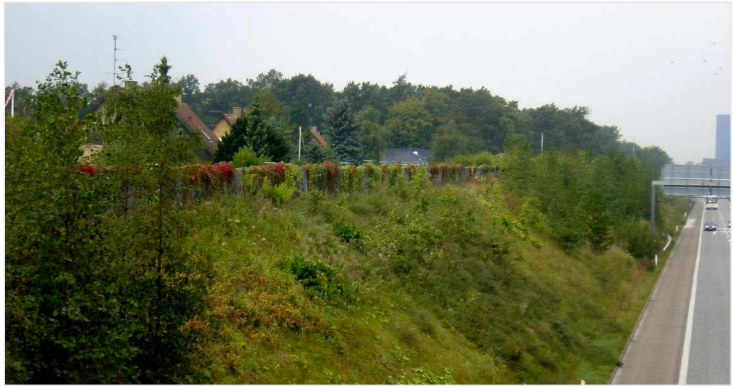
Figure 3.24. Noise barrier with vegetation on top of earth embankment in Denmark [2].
