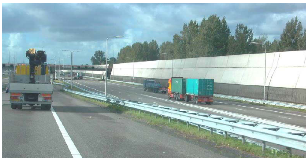
Figure 1.3. Noise barriers can be large structures which have an impact on the local physical environment. Shaped gray and white concrete barrier at a highway in the Netherlands.
