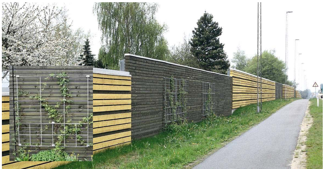
Figure 3.35. Wooden noise barrier with steel net to support vegetation at National Road 310 in Horsens, Denmark (detail to the left).
