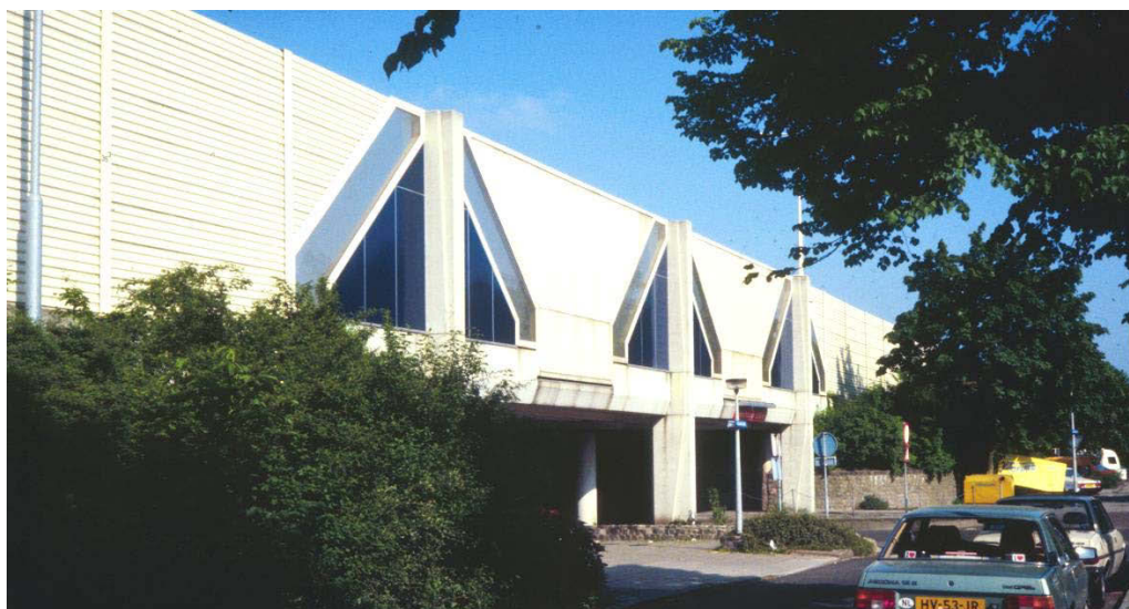
Figure 1.7. 5 m high steel and Plexiglas noise barrier from the Netherlands on a bridge at Highway A9 functioning as a visible addition to its surroundings through a conscious selection of materials, colors and forms [3].
