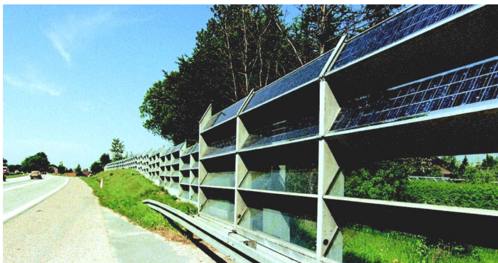
Figure 3.14. Transparent steel noise barrier with electric solar panels at the top. At Highway M11 at Fløng, West of Copenhagen, Denmark [1].
