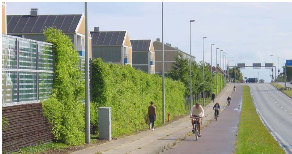
Figure 2.11. Danish transparent noise barrier with vegetation that can reduce the noise reflection.
