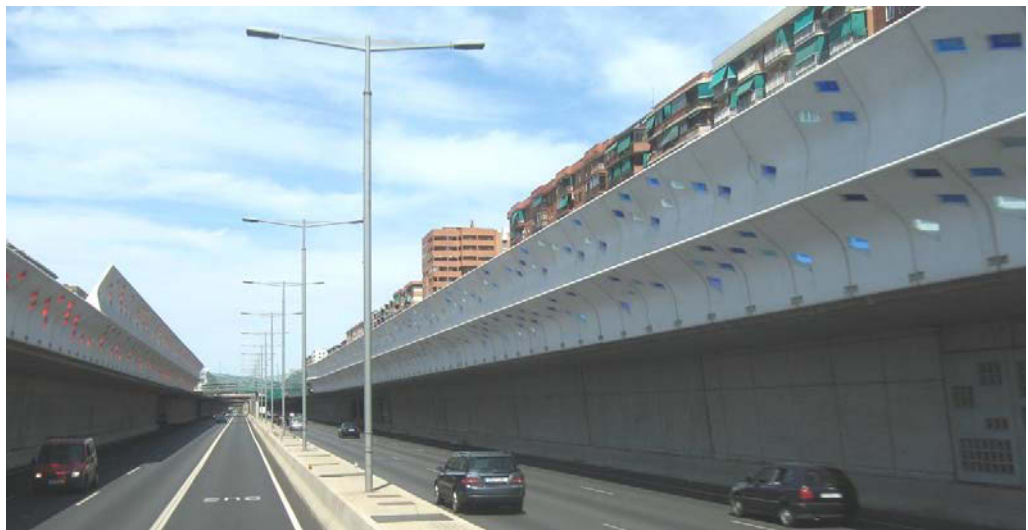
Figure 2.4. Depressed highway partly covered at the road sides and with white concrete noise barriers bending over the highway with colored transparent elements in Barcelona, Spain.
