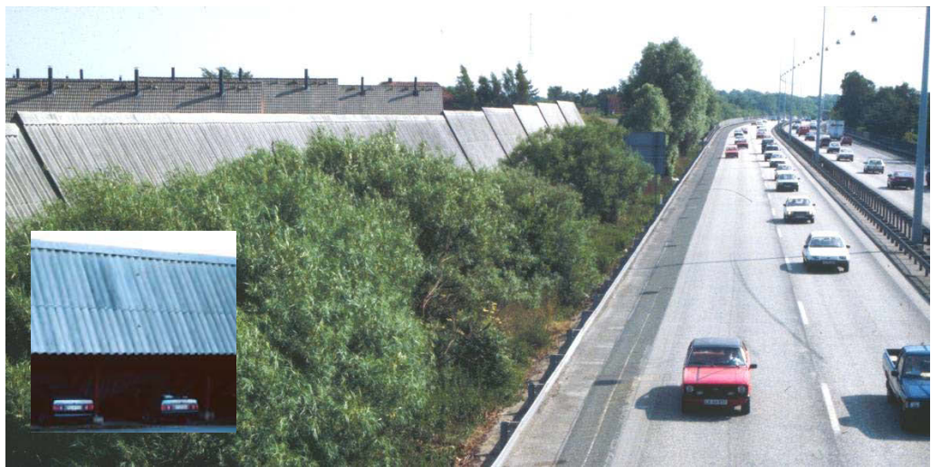
Figure 3.15. The roof of the carport construction for a residential row house area used as a high noise barrier along the M3 ring road around Copenhagen, Denmark [3].
