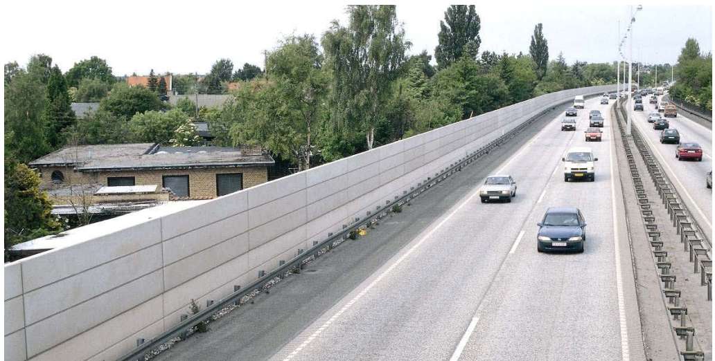
Figure 3.5. Highway side of 3½ m (12 ft) concrete noise barrier in Rødovre along the M3 ring road around Copenhagen, Denmark [1].
