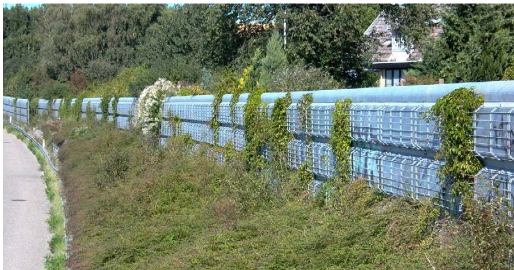
Figure 3.32. Steel noise barrier with steel grid to support vegetation on the barrier at Highway M14 north of Copenhagen, Denmark.
