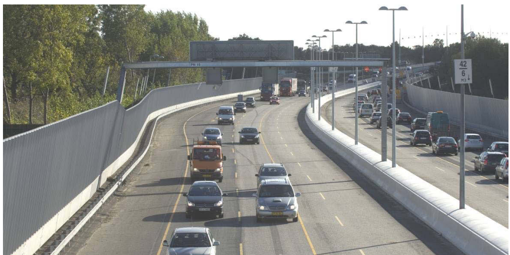
Figure 3.18. 4 m (13 ft) high aluminum absorbing noise barriers bent 10° towards the road along both sides of the M3 ring road around Copenhagen, Denmark (photo Jens V. Nielsen).
