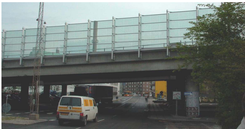
Figure 3.1. Transparent noise barrier designed for use on a highway bridge in an urban environment in Nørrebro, Copenhagen, Denmark.
