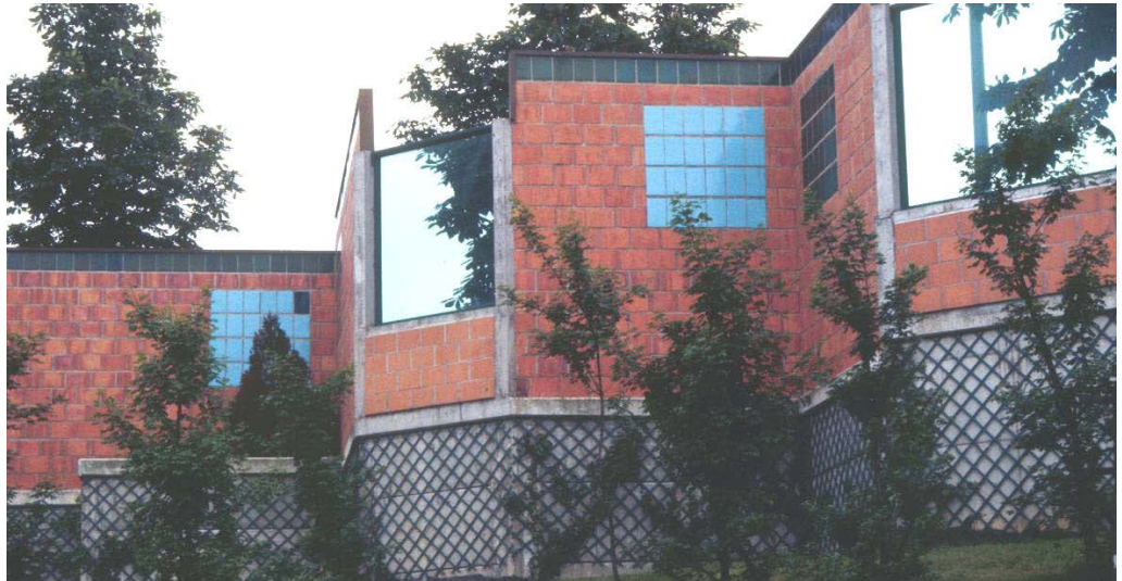
Figure 3.2. Noise barrier constructed of bricks with a lot of details along a highway at an urban residential location in Paris [3].
