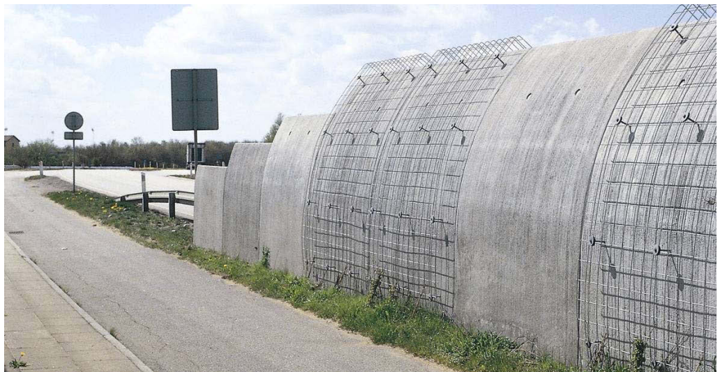
Figure 3.12. Reduced height at the end of a concrete barrier on National Road 411 in Viborg, Denmark [1].
