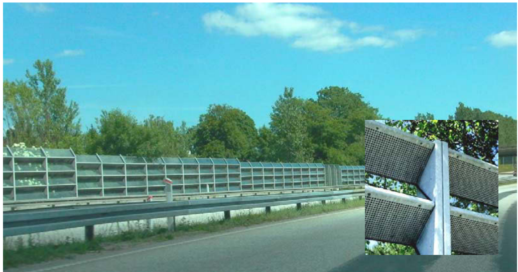
Figure 2.16. 3 to 4 m high transparent steel and glass barrier along Highway M11 near Fløng west of Copenhagen, Denmark [1]. The glass is placed at an angle of 45 ° to reflect the noise up in the air. The bottom sides of the steel elements are noise absorbing, see inserted photo to the right.
