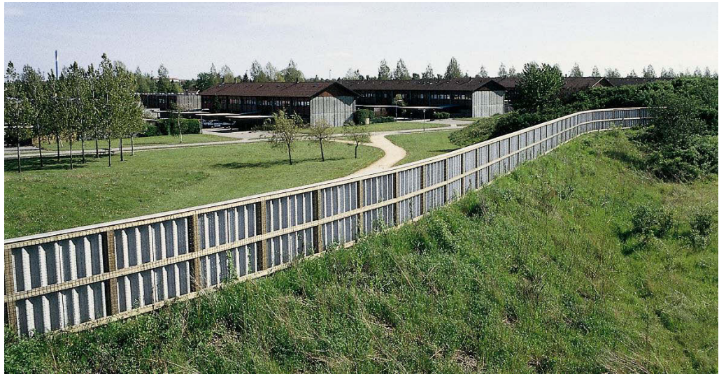
Figure 3.34. 1½ m high eternite (fiber cement) noise barrier with wooden frames on top of an earth embankment at Highway M10 in Greve vest of Copenhagen, Denmark. The barrier has steel net where plants can grow as times goes by [1].
