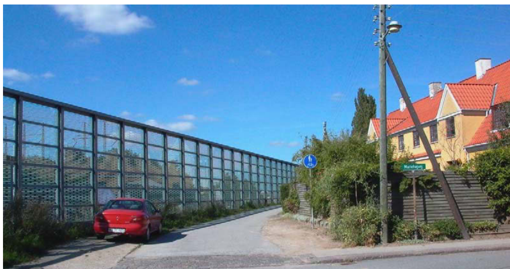
Figure 1.2. Noise barriers have a “back” side facing the nearby town or landscape. Transparent 5 m high noise barrier at Highway M14 north of Copenhagen, Denmark.
