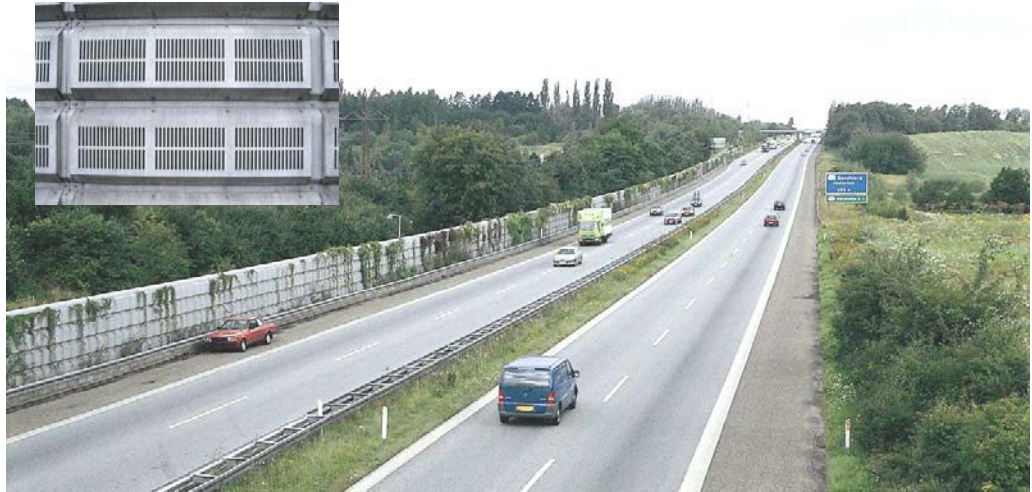
Figure 2.15. 3 to 3½ m high steel noise barrier with absorption elements (see close up to the left) and support for vegetation on Highway M14 north of Copenhagen, Denmark [1].
