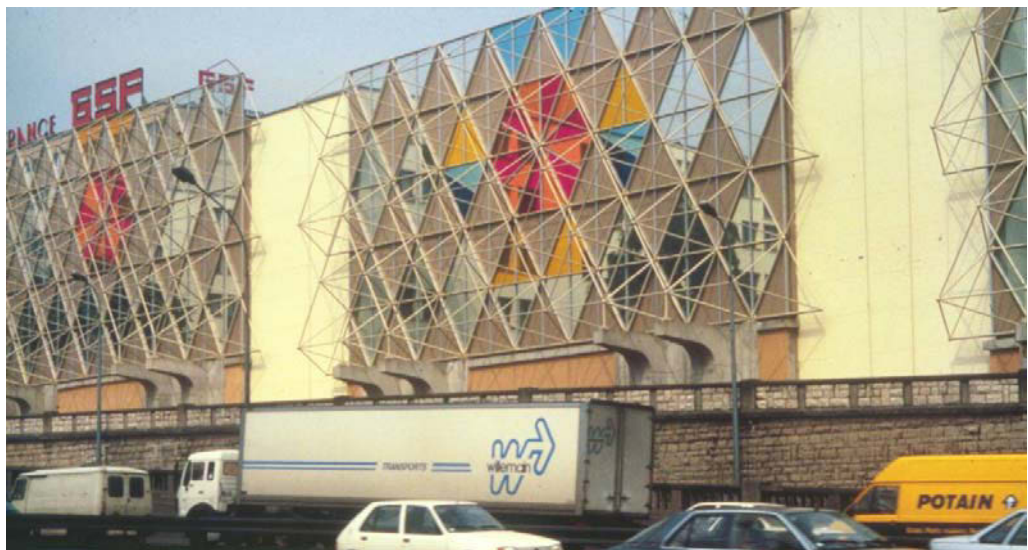
Figure 2.2. 20 m high transparent and colored noise barrier in Paris, France between two 5 story apartment blocks [3].
