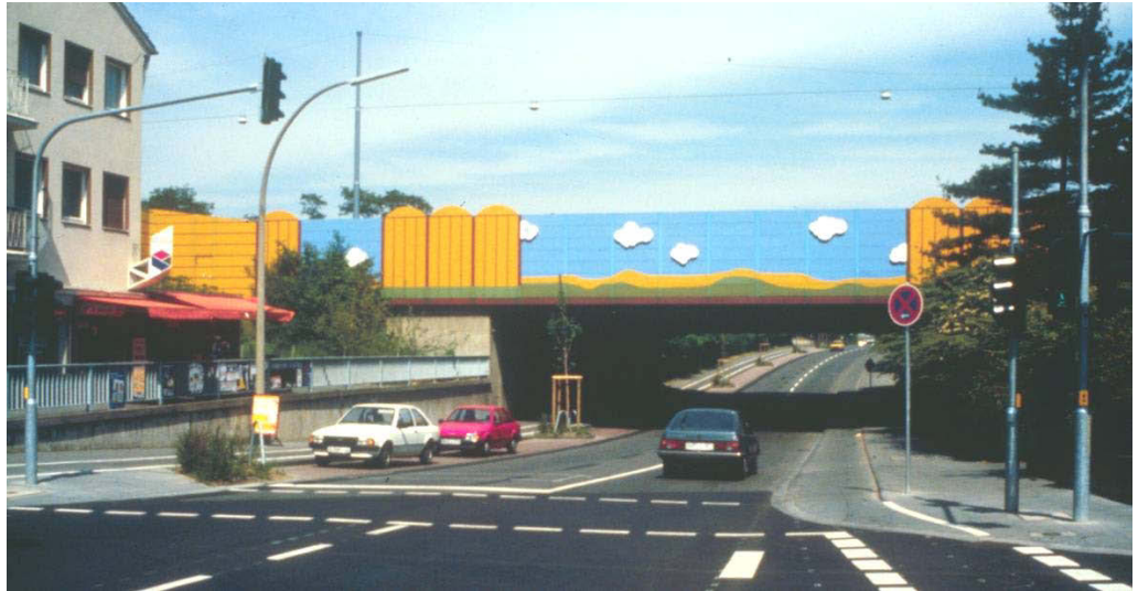
Figure 3.17. Noise barrier as a colorful urban element where Highway 555 in Germany passes on a bridge over a local road [3].
