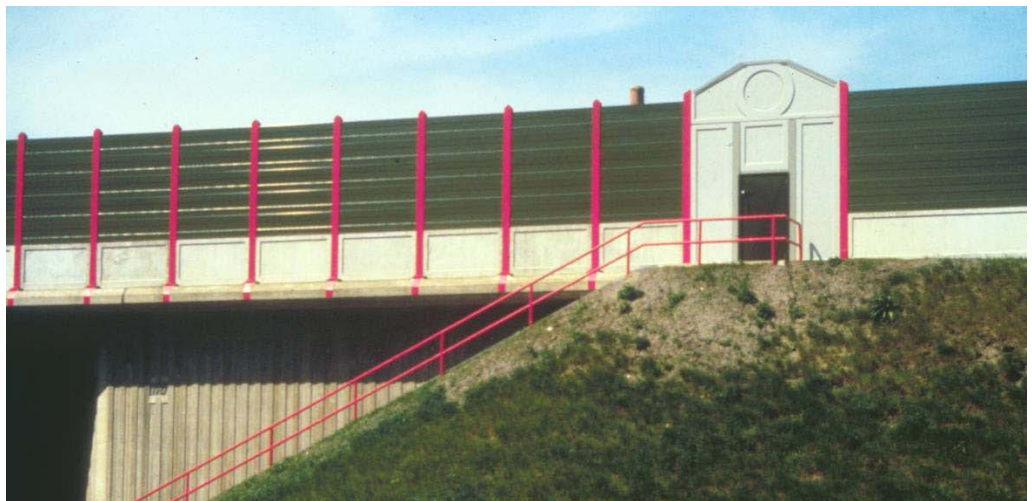
Figure 1.6. 3½ m high dark green steel noise barrier with red steel posts designed using typical building shapes of the surrounding urban environment along a highway south of Hanover, Germany [3].
