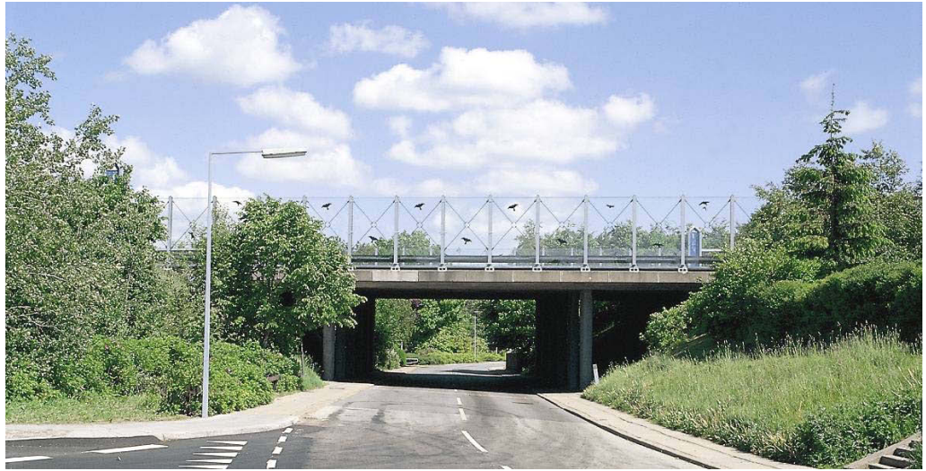
Figure 3.8. Transparent noise barrier used where Highway M70 crosses a local road in Ålborg, Denmark [1]. This allows the drivers on the highway to get a sight of the surrounding landscape.
