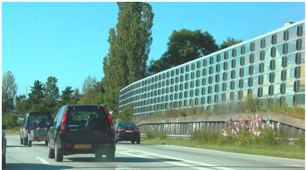
Figure 1.1. Noise barriers have a “front” side facing the highway. Transparent 5 m high noise barrier at a 1½ m high embankment at Highway M14 north of Copenhagen, Denmark.
