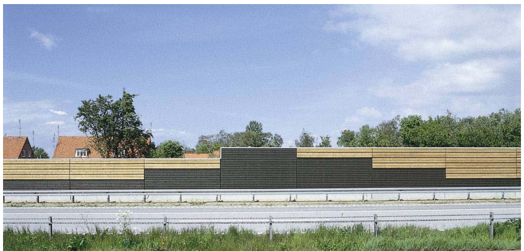
Figure 3.3. 2 to 3 m (6 to 10 ft) high wooden noise barrier at Highway M30 in Saksøbing in Denmark [1].
