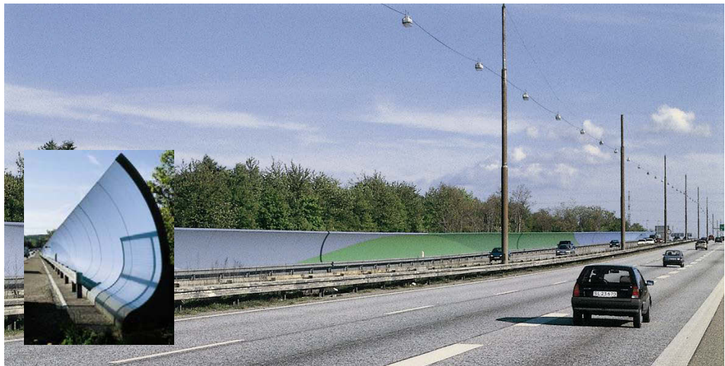
Figure 3.26. 3 m (10 ft) concrete noise barrier constructed in a curved shape and painted along Highway M13 in Gladsaxe north of Copenhagen, Denmark [1].
