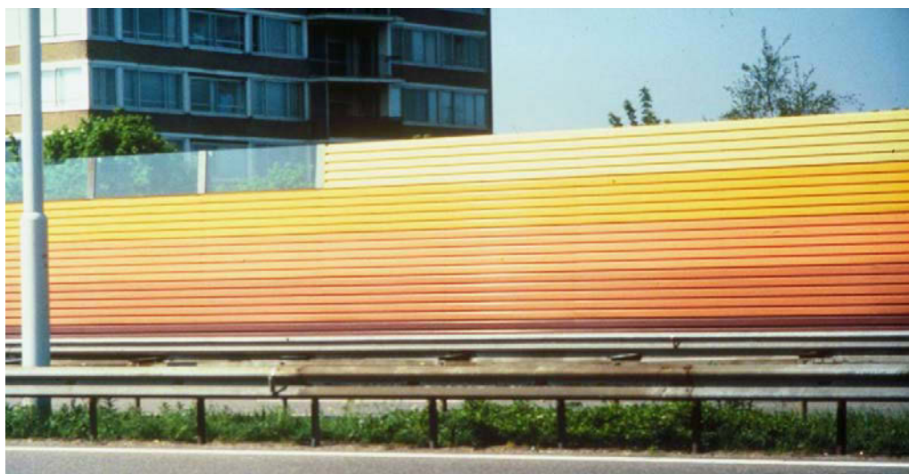
Figure 2.17. 4½ m high colored noise absorbing steel barrier with perforated surface and absorbing material at Highway A9 in the Netherlands [3].
