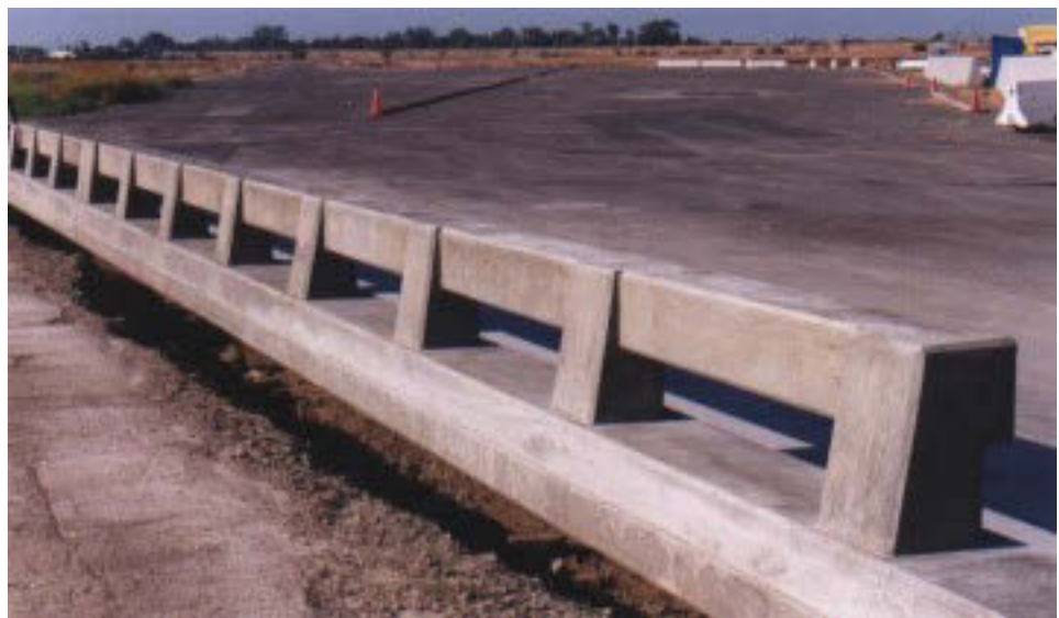
Figure 2-12 Backside of Completed Bridge Rail
