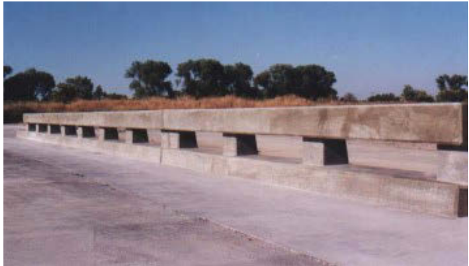
Figure 2-10 Completed Type 80 Bridge Rail
