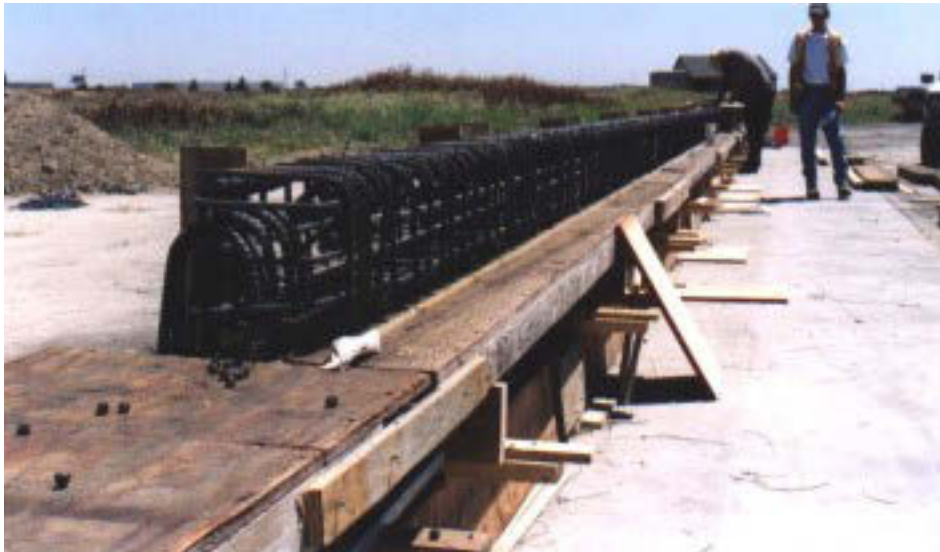
Figure 2-5 Steel Placement for Beam Section
