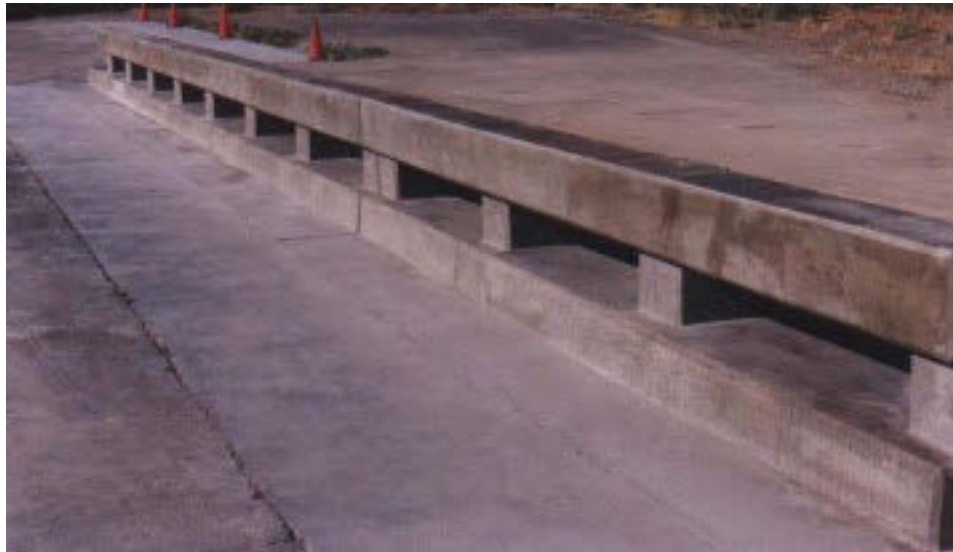
Figure 2-11 Completed Type 80 Bridge Rail
