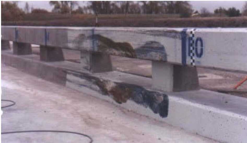
Figure 2-30 Test 545 Impact Area
