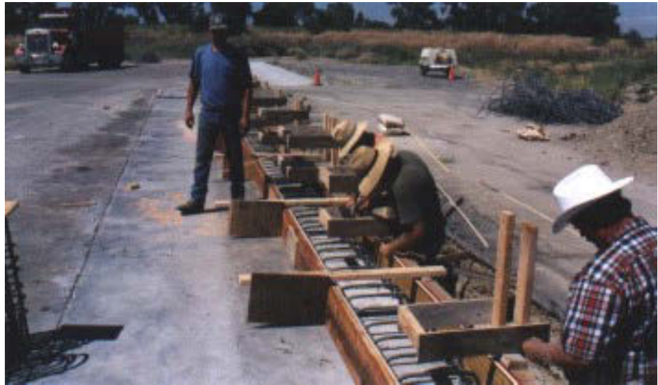
Figure 2-4 Form Construction for Curb
