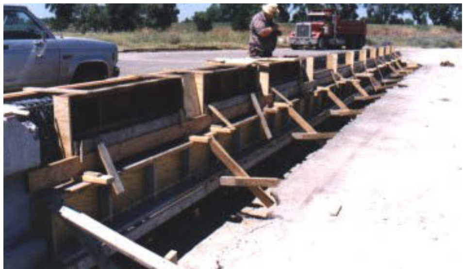
Figure 2-6 Form Placement for Beam Section
