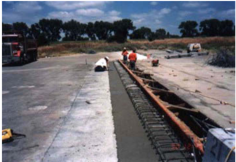
Figure 2-3 Simulated Bridge Deck Construction
