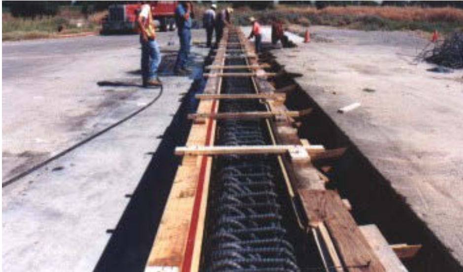
Figure 2-8 Top View of Forms for Beam Section
