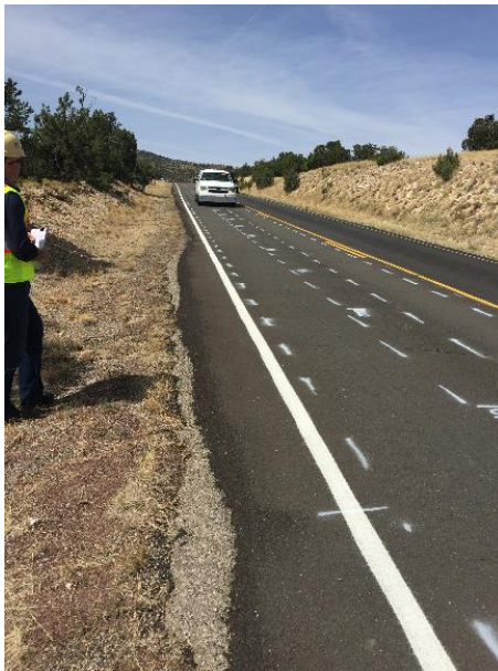
Figure 13. Example of wheel path marking prior to crack survey.
