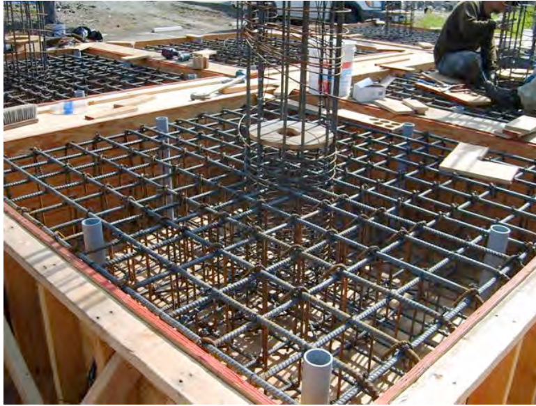
Fig. A.16 Anchor block reinforcement cage.
