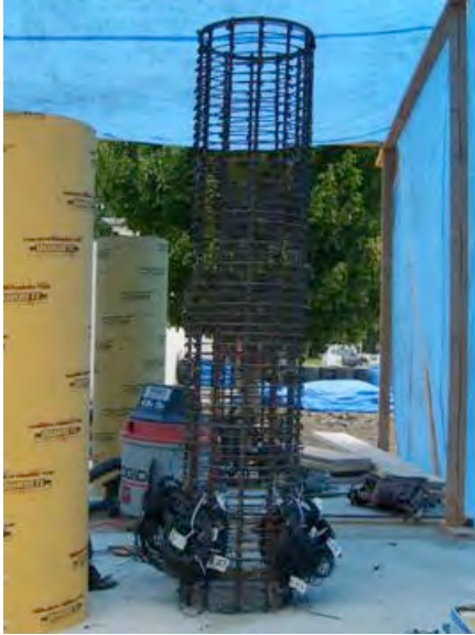
(a) After construction of the column cage
