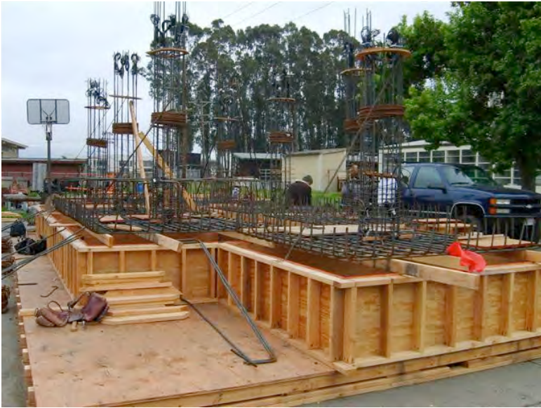
Fig. A.15 Placement of longitudinal bars.
