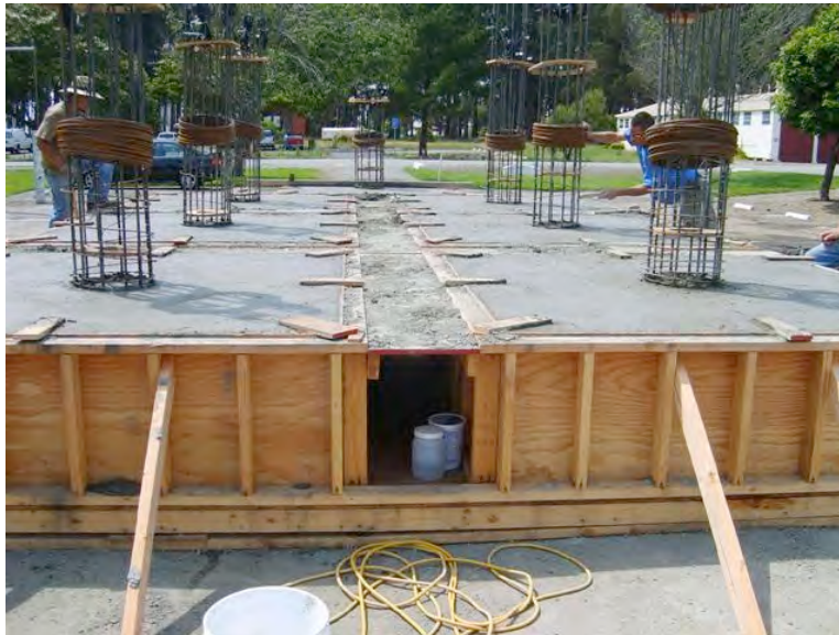
Fig. A.18 After casting the anchor blocks.
