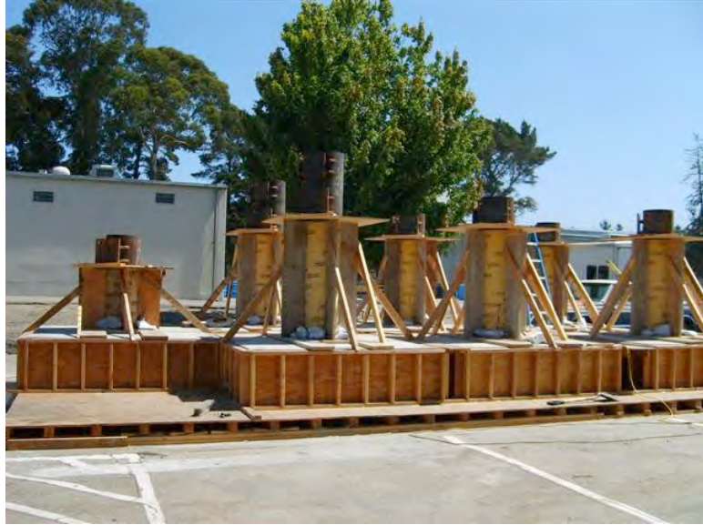
Fig. A.21 Installation of steel jackets.
