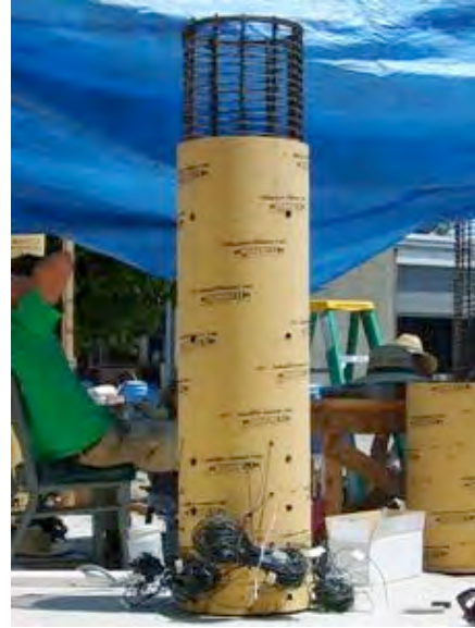
(b) After putting the Sonotube
