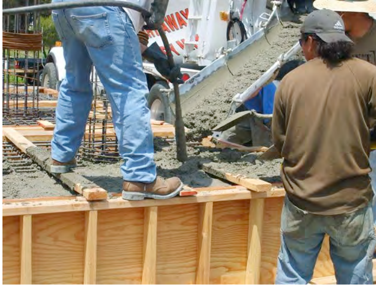
Fig. A.17 Casting anchor block.
