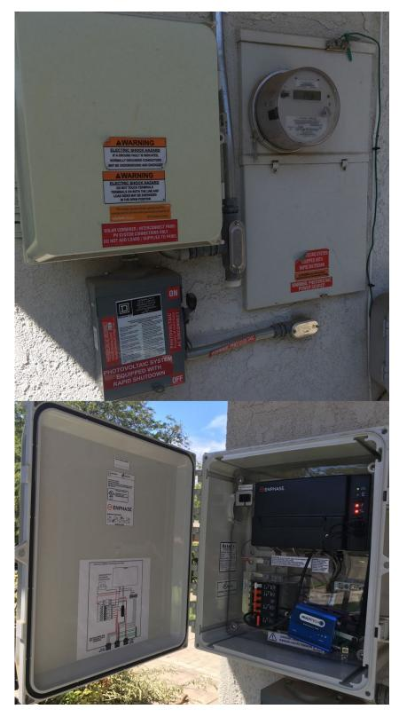
Figure 6.22. Modern interconnect for system with microinverters. Photo credit: Kurtz.
