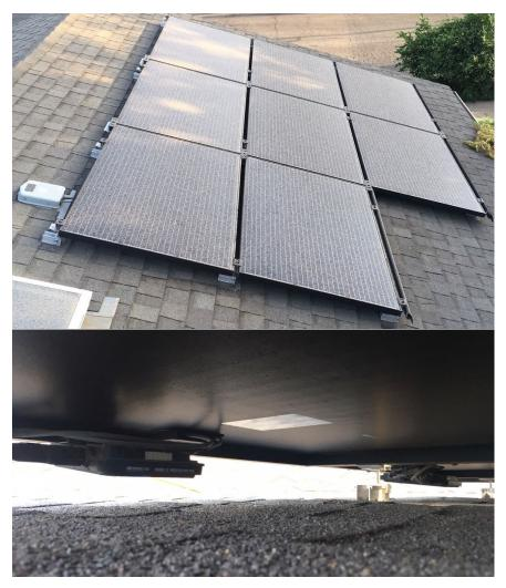
Figure 6.21. System with microinverters (top); microinverter between module and roof (bottom). Photo credit: Kurtz.
