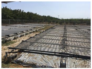
Figure 6.5. Deployed CIGS system by Solyndra. Photo credit: Kurtz.
