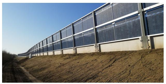
**Figure 3.1. Bifacial modules for noise barriers.** Image source: Solar Energy Application Centre, https://www.pv-magazine.com/2019/02/20/bifacial-modules-ridin-down-the-highway/.
