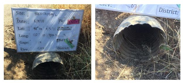
Fig. 3.4 Left: a culvert with a score of 3, Right: a closer look at the invert
