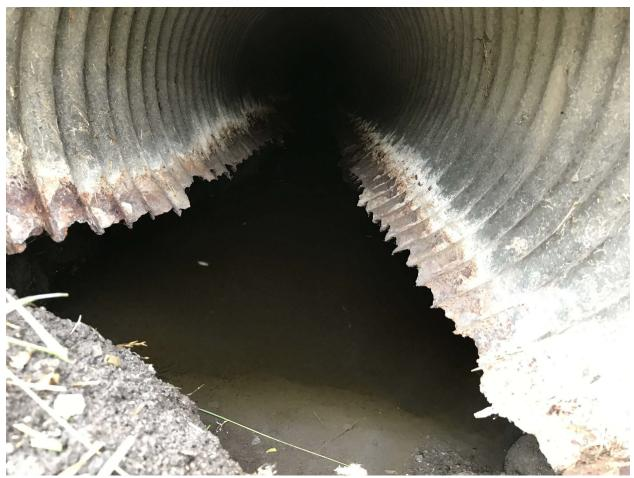
Fig. 3.7 A culvert from a coastal highway in San Luis Obispo County with severe corrosion due to high salinity
