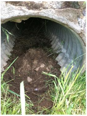
**Fig. 3.8** A Forest land culvert (heavy water flow has filled the culvert; however, very little corrosion has resulted from this due to non-corrosive soil environment)
