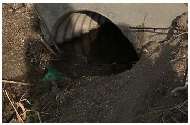
Fig. 3.2 Low slope accumulates standing water due soil at culvert outlet
