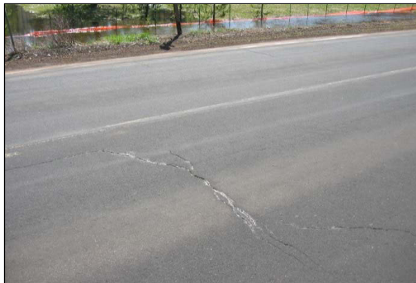
Figure 2.1: Transverse crack.
