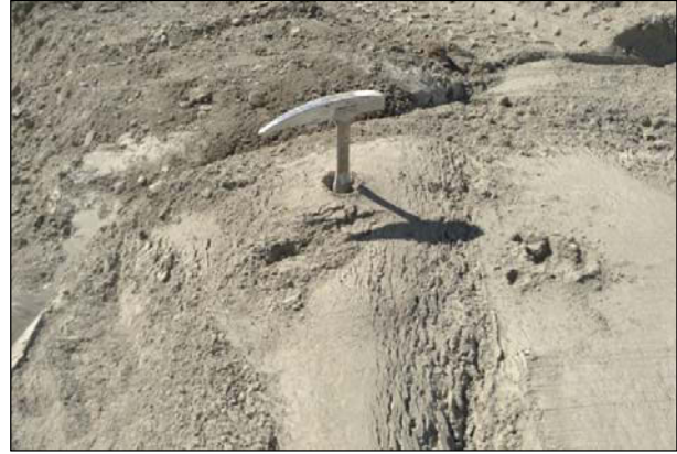
Figure 3.21: PLU147: Depth of cement mound due to dragging of hose ( \pm 200 mm).
