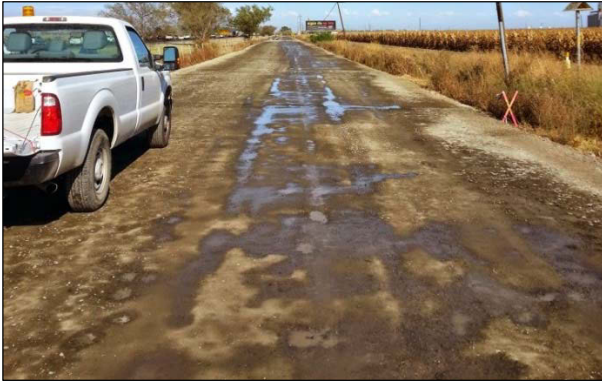
Figure 3.5: CR32B: Surface raveling.
