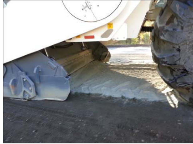
Figure 3.22: Wave of cement in front of pulverizer skirt on mixing chamber.
