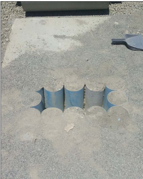
Figure 5.5: Test pit preparation.
