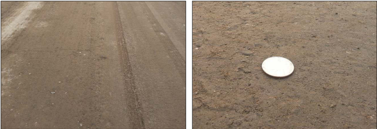
Figure 3.10: CR27: Fine graded material near start of project.
