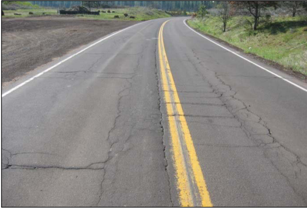
Figure 2.3: Block cracking.
