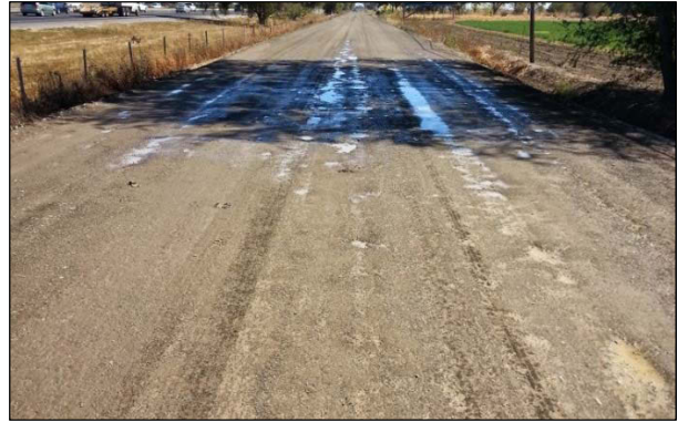
Figure 3.5: CR32B: Surface raveling.
