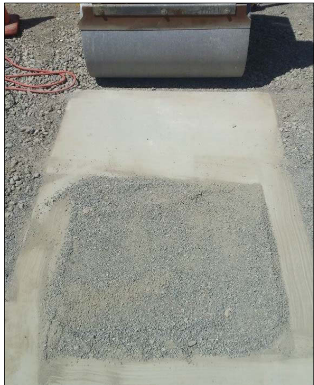
Figure 5.6: Final setup before microcracking.
