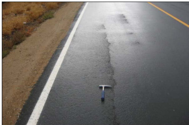
Figure 2.2: Longitudinal crack.
