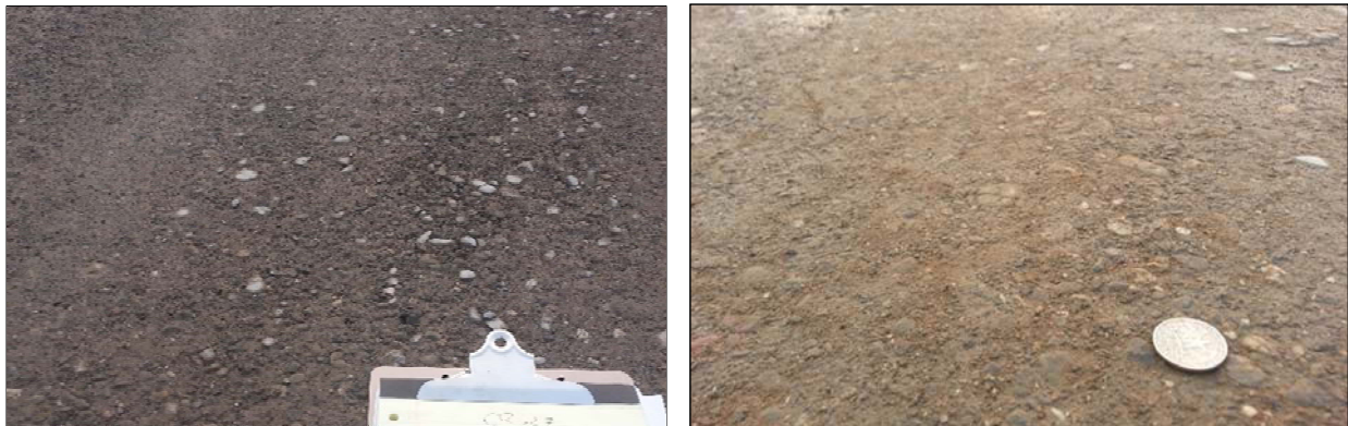
Figure 3.11: CR27: Coarser material throughout majority of the project.
