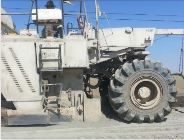
Figure 3.22: Wave of cement in front of pulverizer skirt on mixing chamber.
