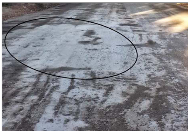
Figure 3.8: CR32B: Wet section after repair.
