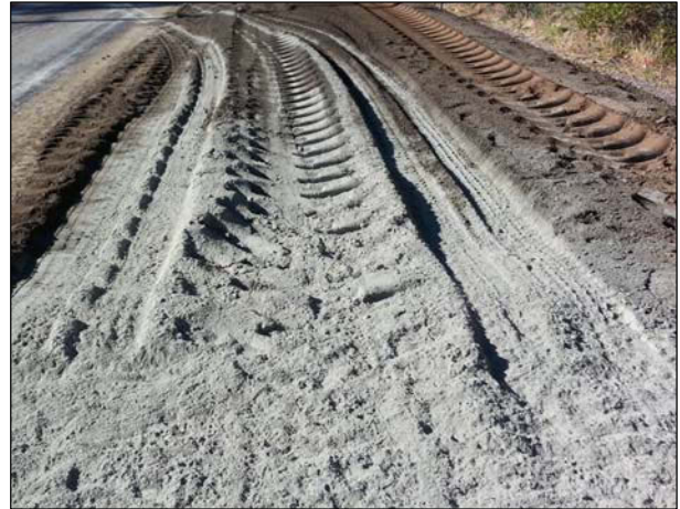
Figure 3.24: Cement spreader spreading cement on already mixed section.
