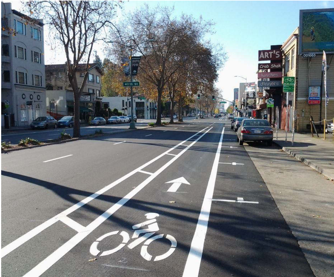
Figure 2: Example of Class II Facility: Broadway, Oakland
