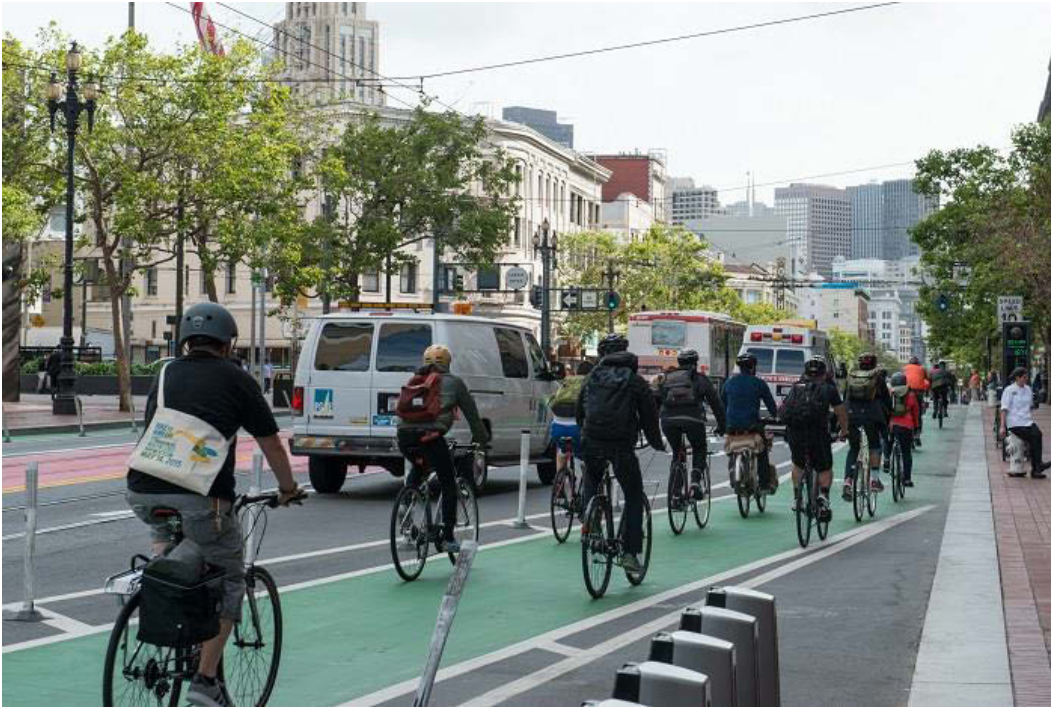
Figure 4: Example of Class IV Facility: Market Street, San Francisco
