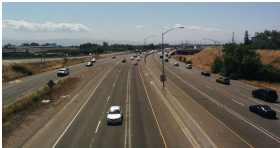
(b) Looking toward westbound
