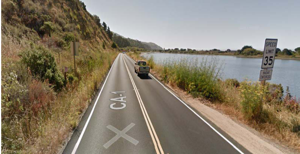
Figure 6.9. PCH-1, 35MPH, Street view, 7-10ft of clear zone because of the speed limit
