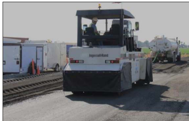
Figure 3.26: FDR-FA: Final compaction showing tightly bound surface.
