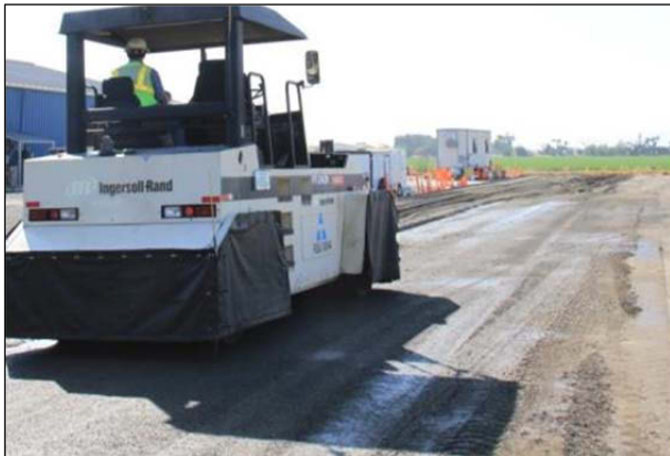
Figure 3.12: FDR-NS: Compaction with rubber-tired roller.
