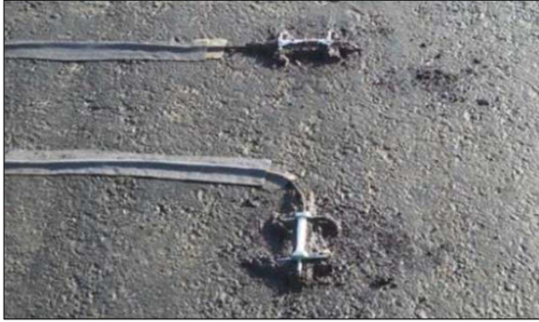
Figure 4.3: Strain gauge installation.
