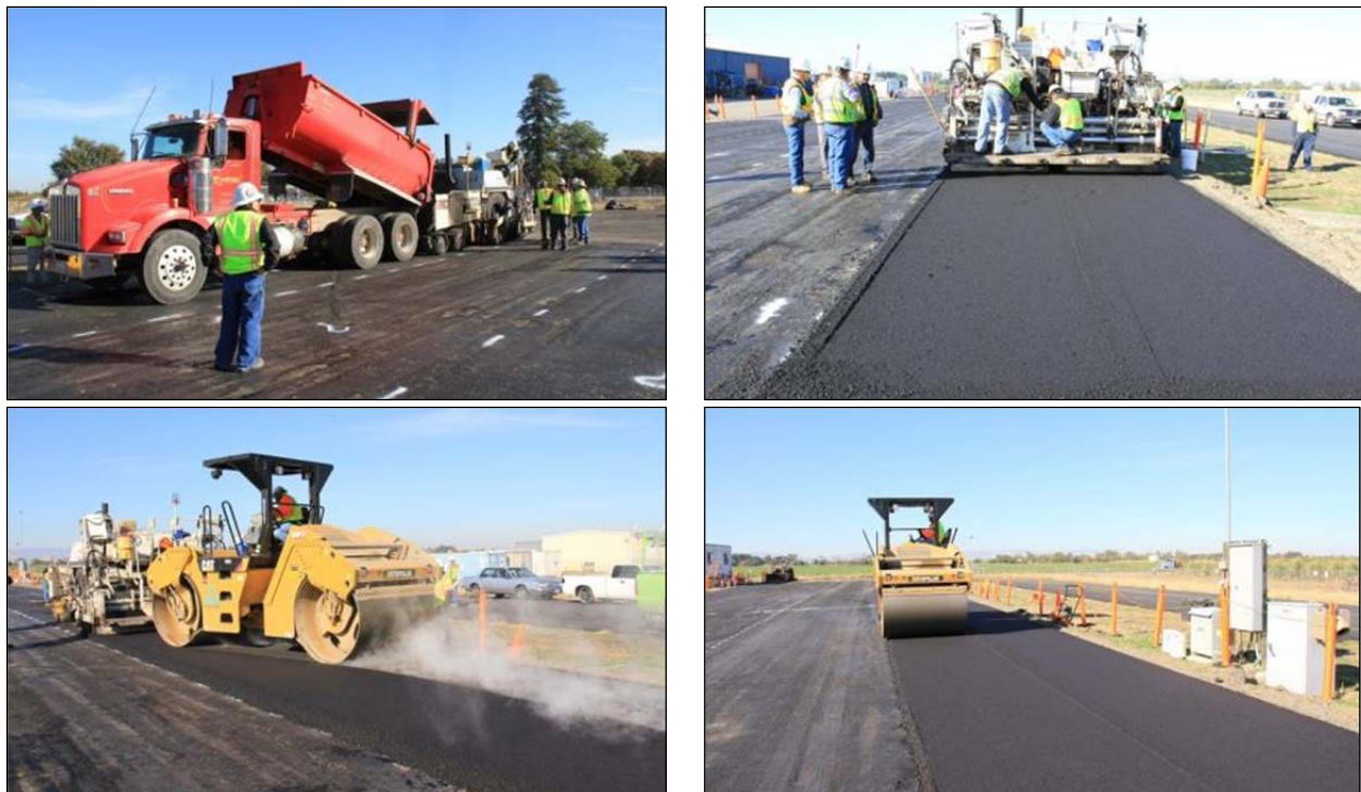
Figure 3.37: Asphalt concrete placement.
