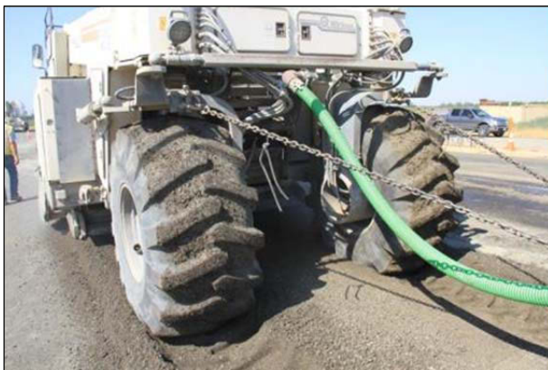
Figure 3.23: FDR-FA: Uniform mix behind recycler.
