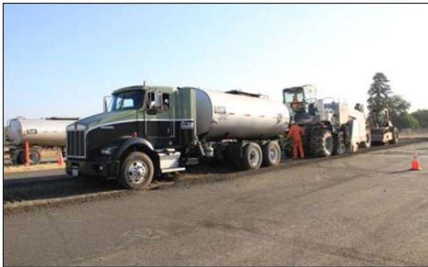
Figure 3.14: FDR-EE: Recycling train.
