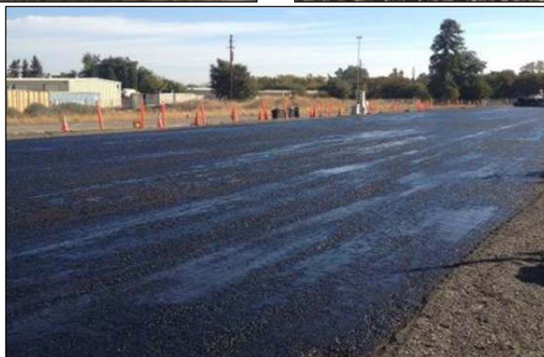
Figure 3.36: Prime coat application.
