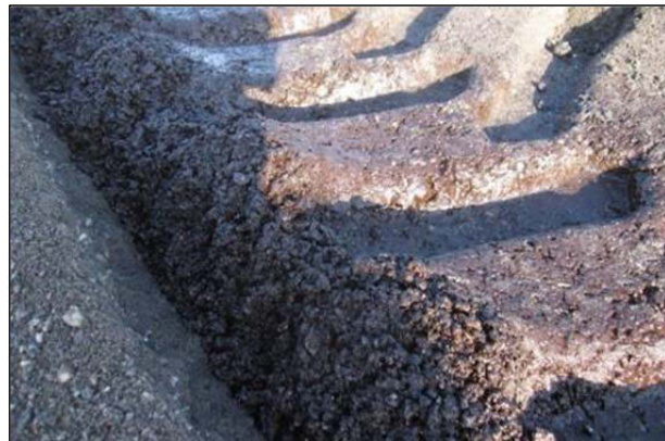
Figure 3.16: FDR-EE: Excess emulsion applied during recycling.
