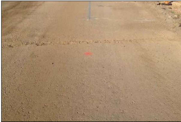
Figure 3.34: Broomed surface of FDR-NS layer.
