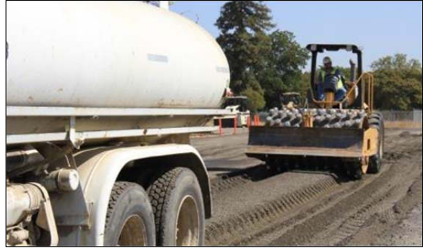
Figure 3.9: FDR-NS: Initial compaction with padfoot roller.
