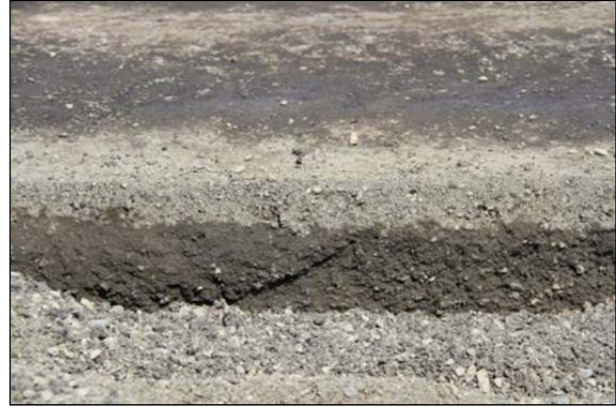
Figure 3.20: FDR-EE: Excavation showing wet recycled layer.
