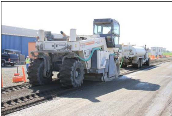
Figure 3.31: FDR-PC: Second mixing pass with water.
