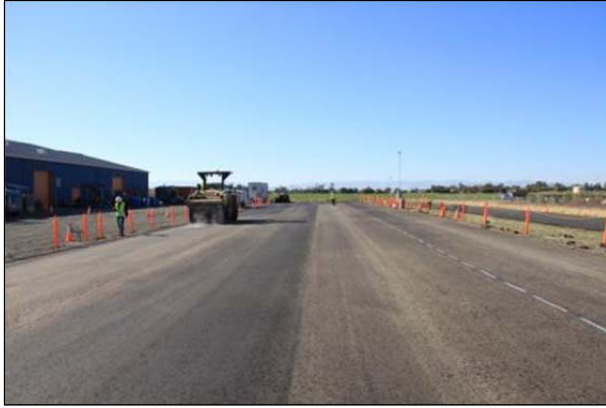
Figure 3.38: First lift of asphalt concrete after compaction.
