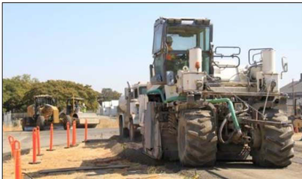
Figure 3.5: FDR-NS: Test track recycling.
