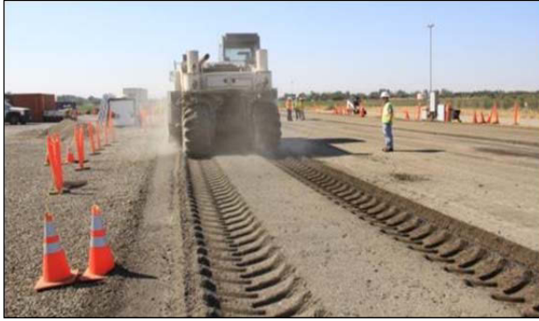
Figure 3.29: FDR-PC: Uniform mixing after first pulverization pass with no water.
