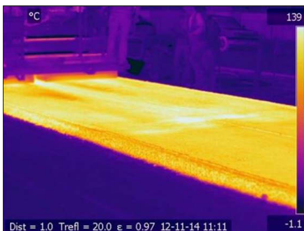
Figure 3.40: Thermal image of test track during construction.
