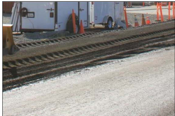
Figure 3.32: FDR-PC: Uniform mix after second recycling pass.
