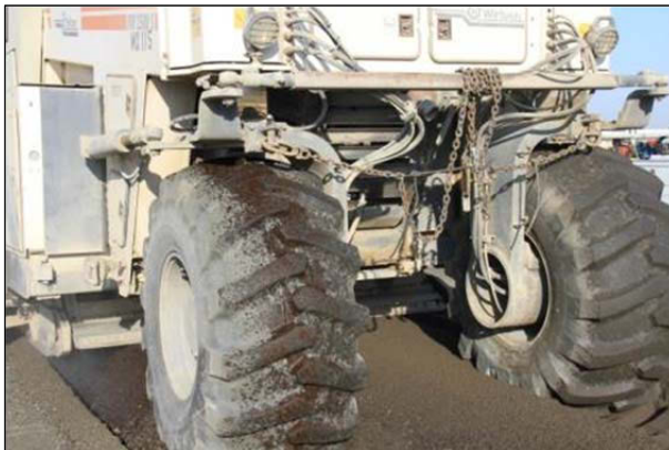
Figure 3.16: FDR-EE: Excess emulsion applied during recycling.
