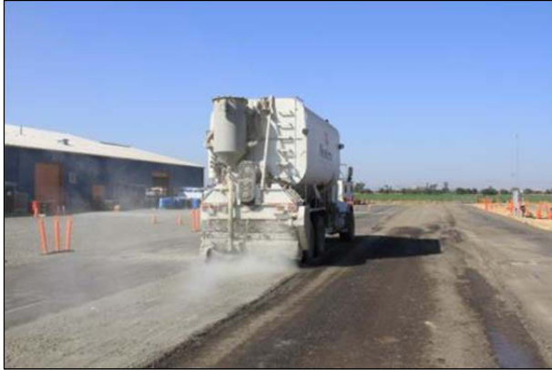
Figure 3.21: FDR-FA: Spreading cement on old asphalt surface.
