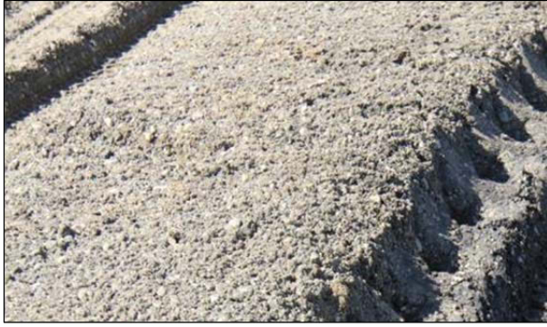
Figure 3.8: FDR-NS: Pulverized material.
