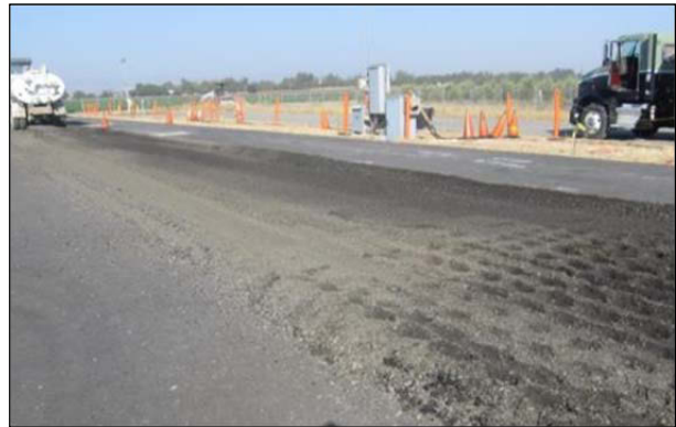
Figure 3.17: FDR-EE: Compaction with padfoot roller. (Note untreated areas and emulsion adhering to tire).
