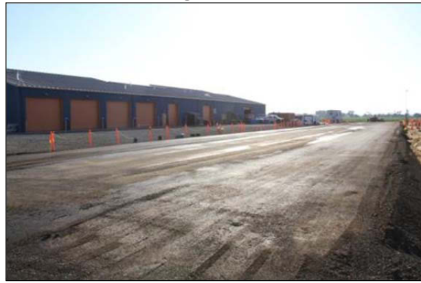
Figure 3.13: FDR-NS: Completed recycled layer surface.
