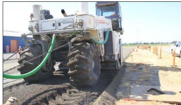
Figure 3.5: FDR-NS: Test track recycling.
