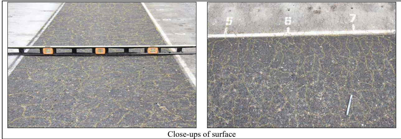
Figure 7.25: 684HB: Test section photographs ( continued ).
