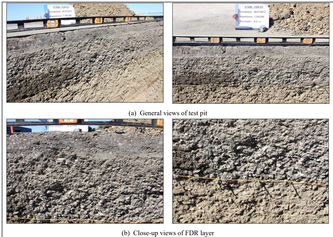
Figure 8.4: 673HB: Test pit photographs.
