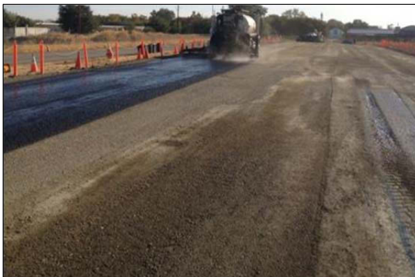
Figure 3.34: Broomed surface of FDR-NS layer.
