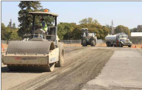
Figure 3.10: FDR-NS: Compaction with smooth drum roller.
