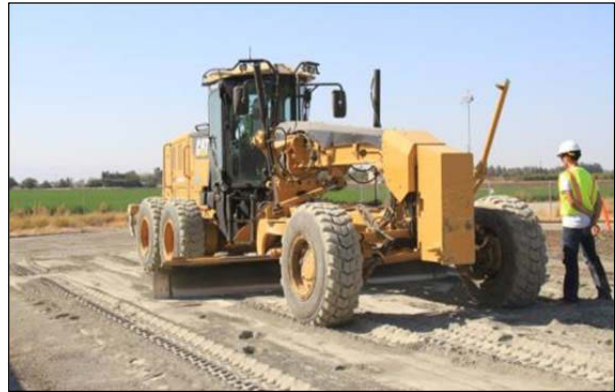
Figure 3.28: FDR-PC: Removing excess cement on Cell #8.
