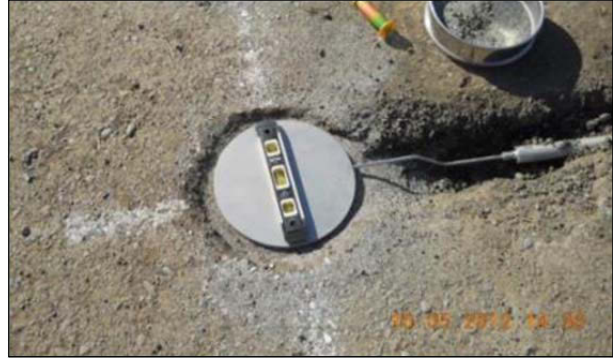
Figure 4.4: Pressure cell installation.
