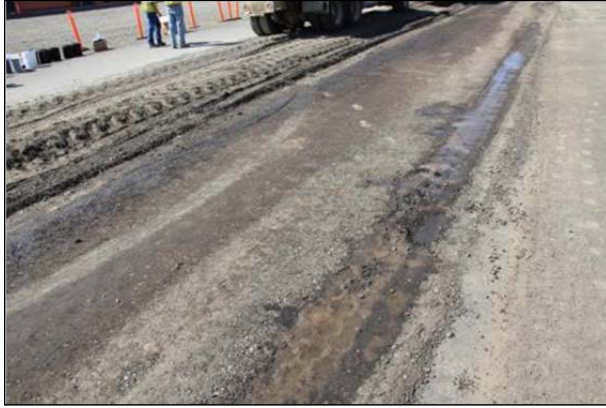
Figure 3.19: FDR-EE: Puddled water on surface after compaction.
