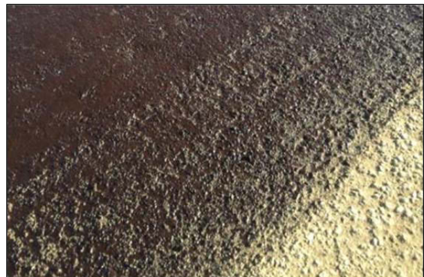
Figure 3.35: Broomed surface of FDR-EE layer showing dark, moist surface.
