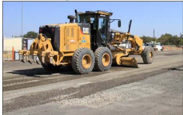
Figure 3.11: FDR-NS: Surface leveling with a grader.
