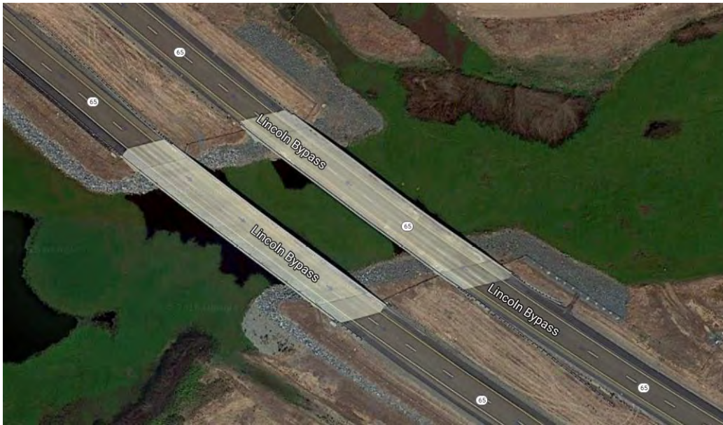
Figure 4.2: Aerial view of Markham Ravine Bridge deck (image acquired from Google Maps)
