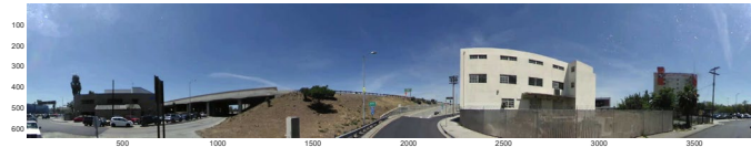
(c) Merging ramp at the entrance of I110N freeway
