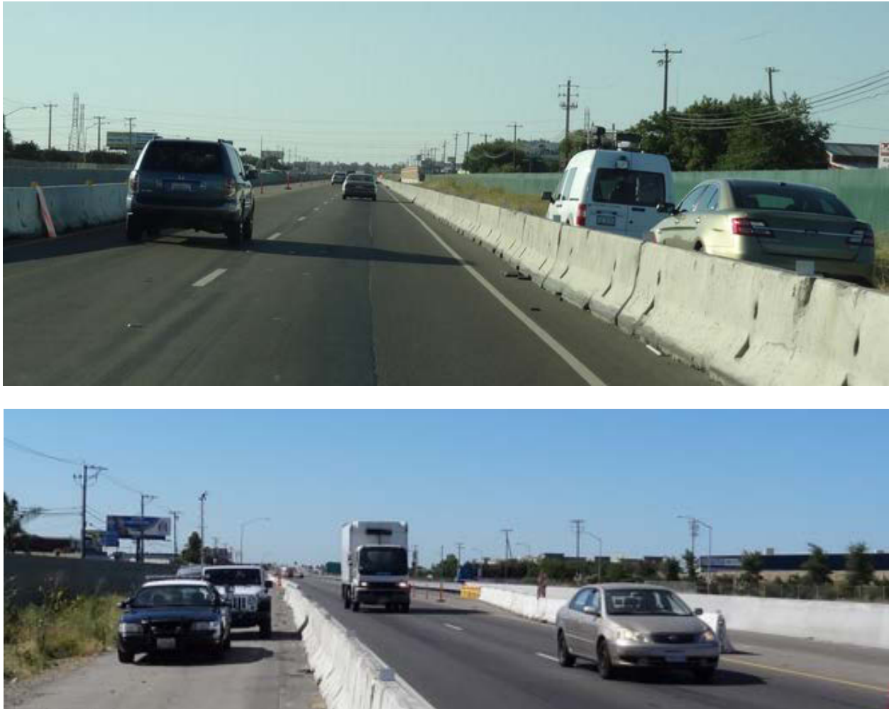
Figure 31. Placement of PSE in Stockton Showing Minimum Distance to Traffic.
