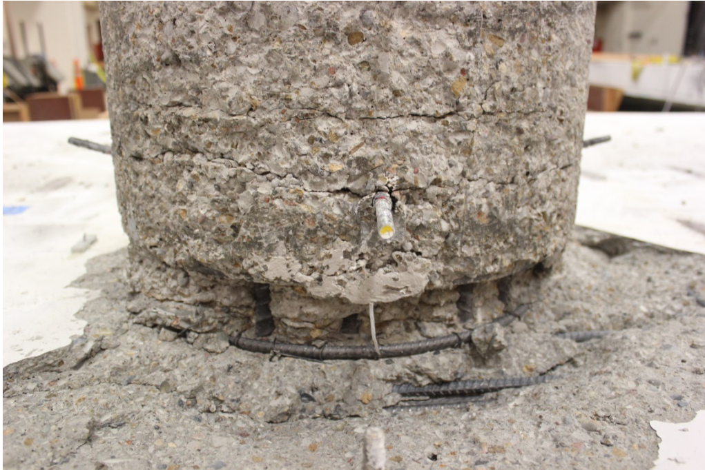
Figure 3.9 A close-up view of Specimen No. 2 column flexural cracks (CFRP jacket was removed) and bent cap beam concrete cover spalling after HS tests.
