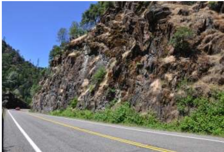
Figure 15. Westbound view of the California SR 299 highway cut.
