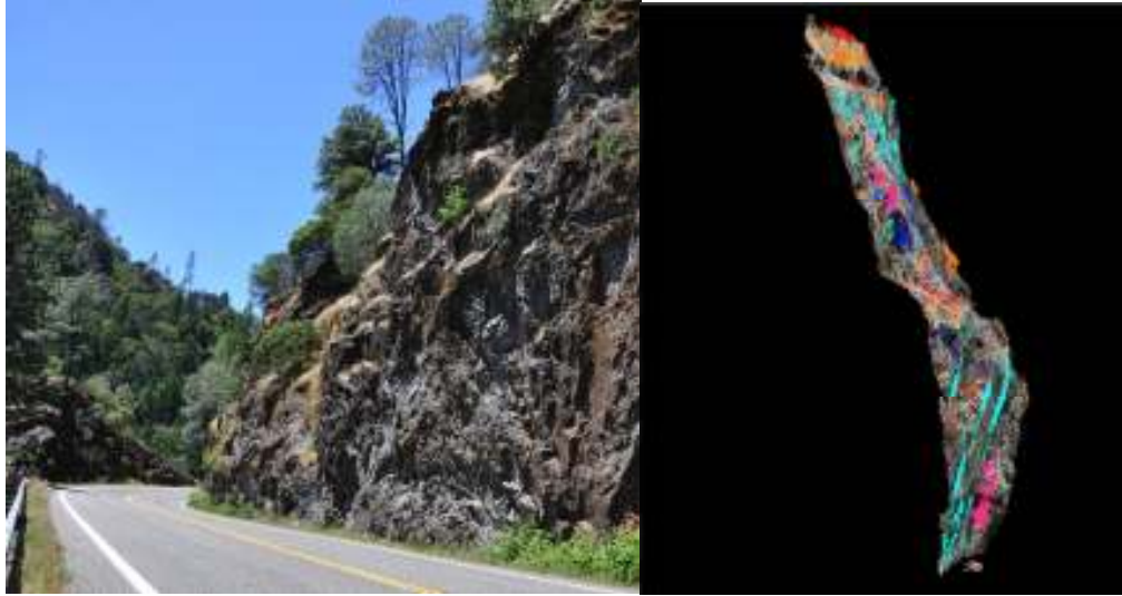
Figure 24. Left to right, a digital image of overhanging fractures of Joint Set 5 (teal) with minimal ditch width, and an image of color point cloud showing overhanging fractures of Joint Set 5 (teal).
