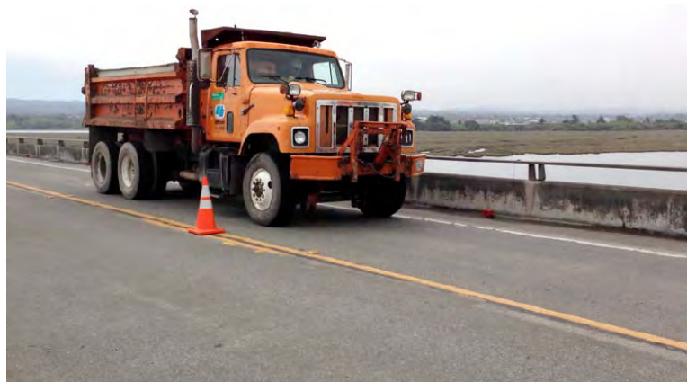
Figure 3-7: Truck test #3 (truck came to a full stop at the center of the middle span within a few yards from 40 mph).
