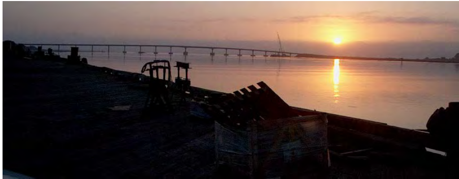
Figure 1-1: Samoa Bridge as viewed from Vance Avenue on the Samoa Peninsula.
