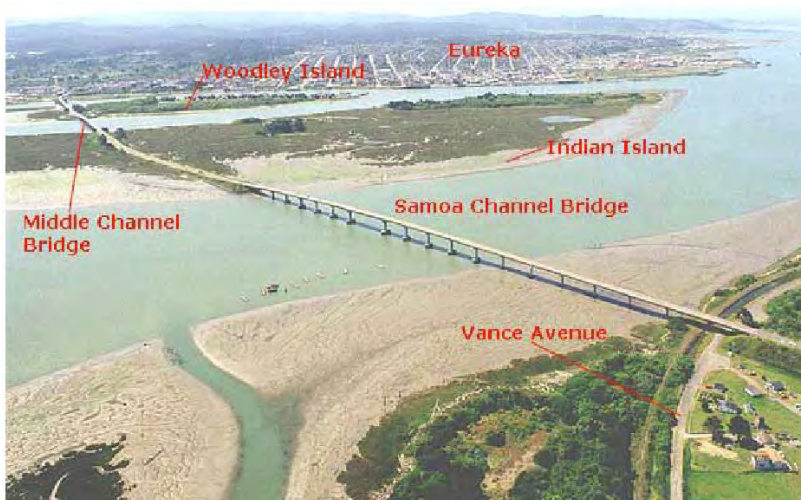
Figure 1-2: General view of the Samoa Bridge.
