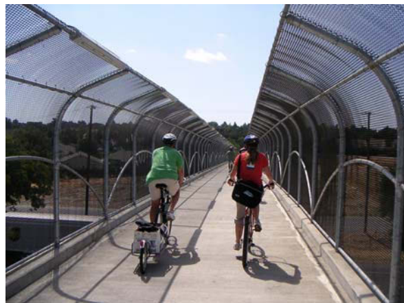
Bicyclists using an overcrossing
