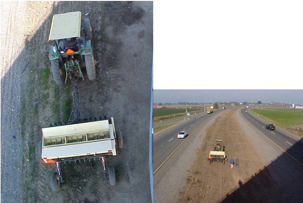
Figure 4. Drill seeding operation at I-5 North on November 23, 2004.
