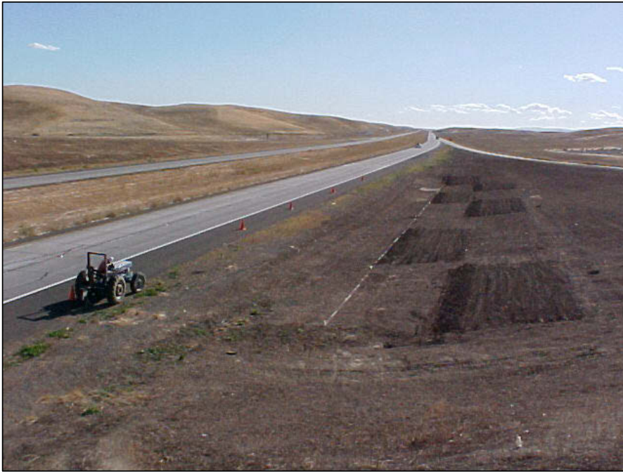
Figure 9. Ripping and cultivation at I505, Yolo County, CA (October 2003).
