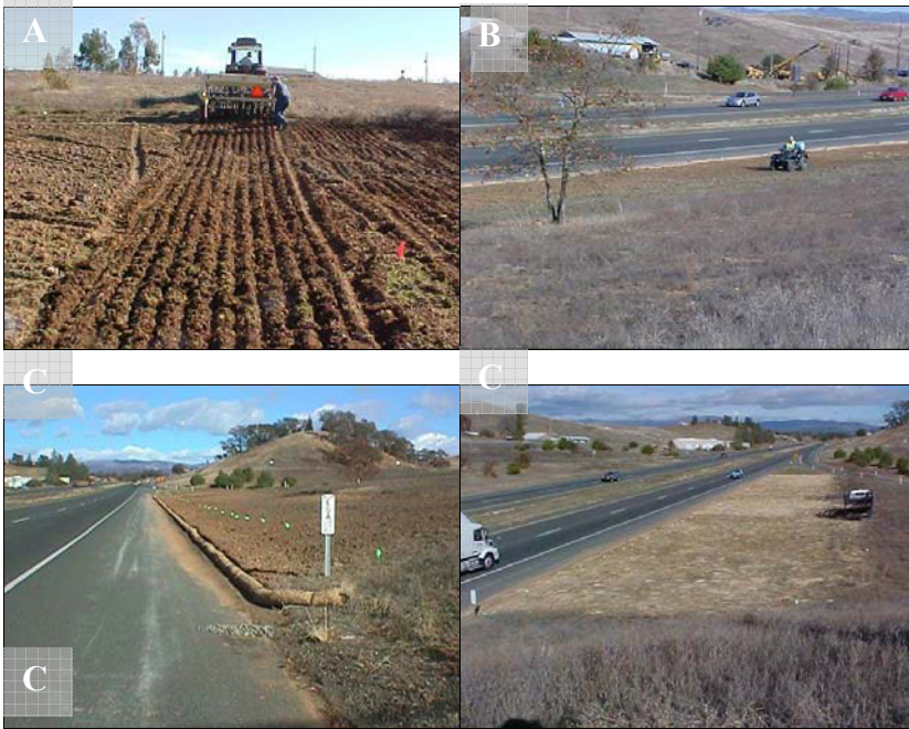
Figure 14. SR29 was drill seeded with native perennial grasses (A), sprayed with glyphosate to control weeds before native grasses emerged (B) and covered with straw to control excessive soil loss across the site and along the road edge (C) (November 2003).
