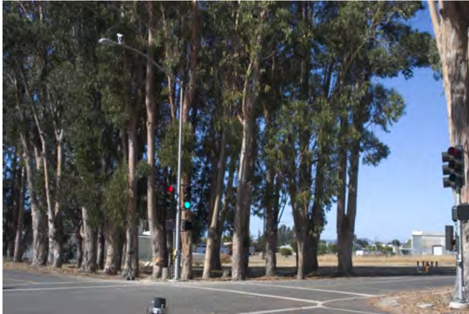
Figure 11. Traficon Video Camera at PATH RFS Intelligent Intersection
