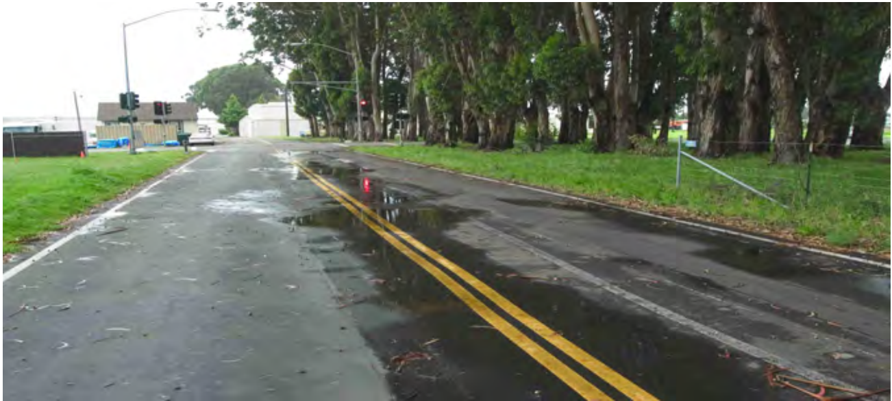
Figure 13. PATH Testbed with Standing Water
