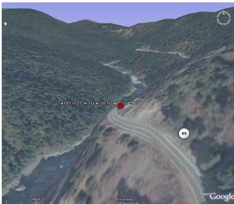
Figure 8: SR 96 Landslide Location - Image Courtesy of Google Earth
