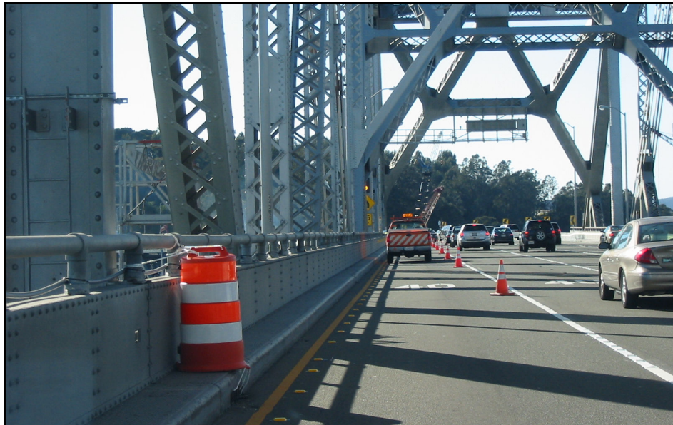
Figure 5. PTMD Installation on the Bay Bridge
