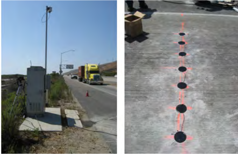
Figure 3-21 Wireless magnetometer setup at upstream station
