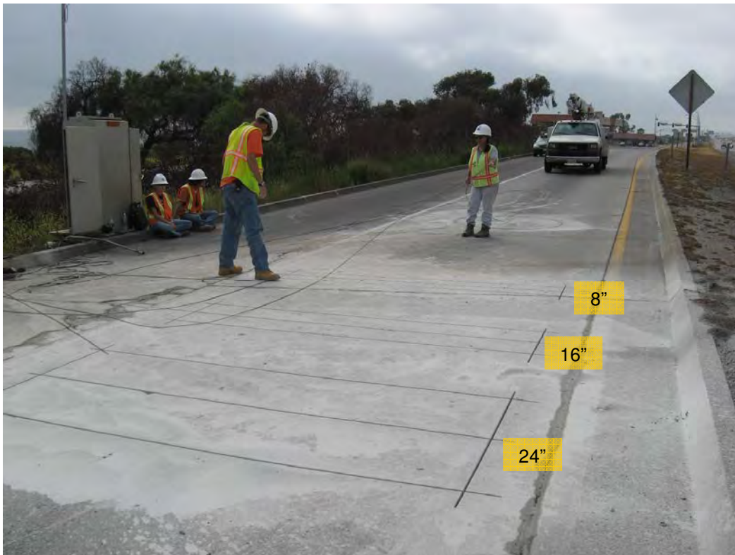
Figure 3-9 Installation of Permanent Blade Sensors
