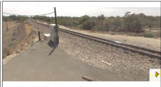
Track View 4: E of crossing, looking S
