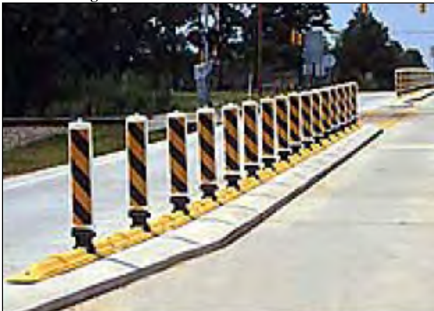
Figure 10: Island Mounted Channelization
