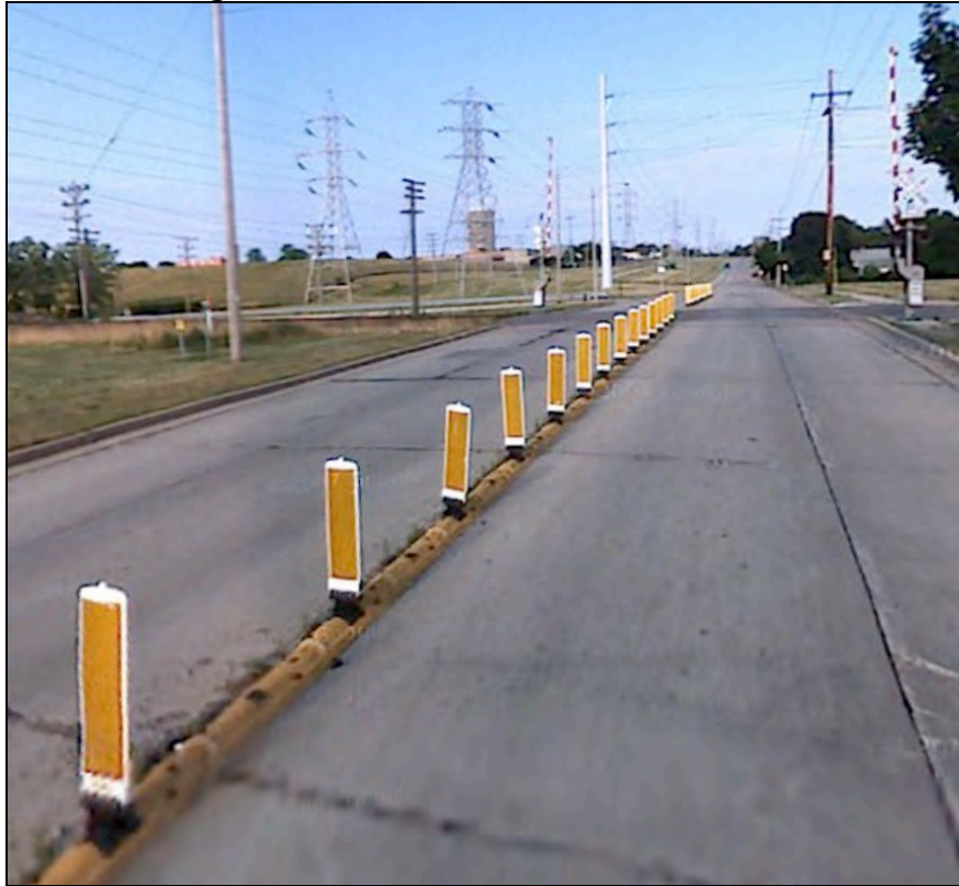
Figure 9: Street Mounted Channelization
