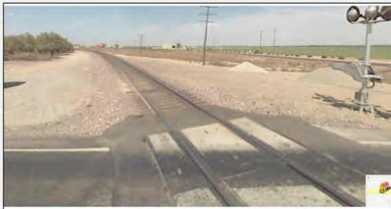
Track View 2: E of crossing, looking N
