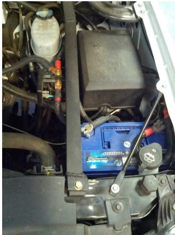
Figure 2.5. Extra battery and battery isolators with circuit breakers added in the engine compartment
