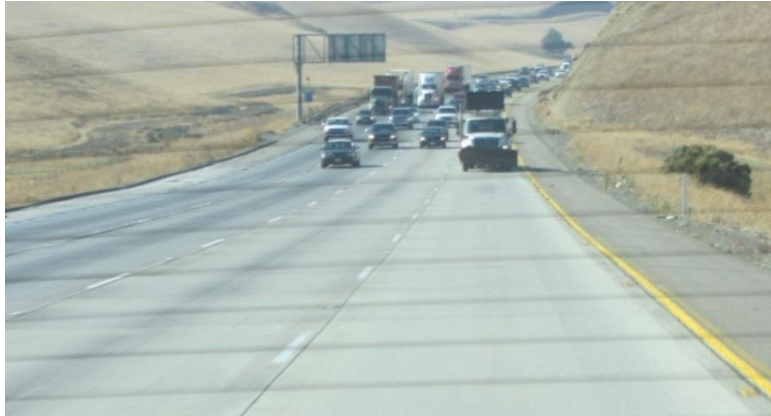
Figure A.5. CHP and shadow vehicle rolling traffic break
