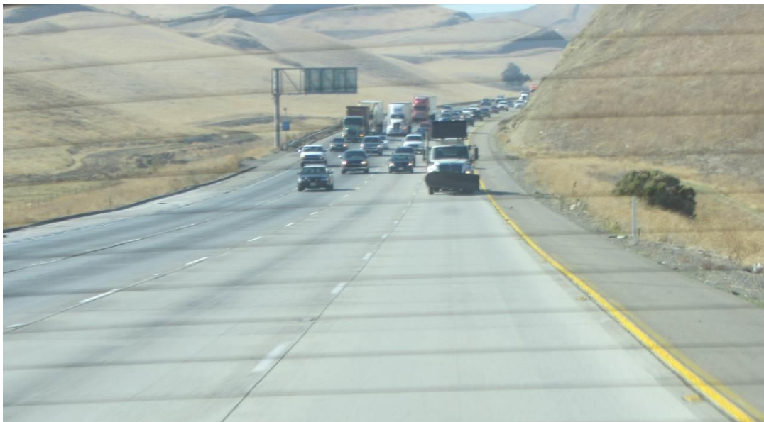
Figure 5.7. Rolling lane closure using CHP and a shadow vehicle
