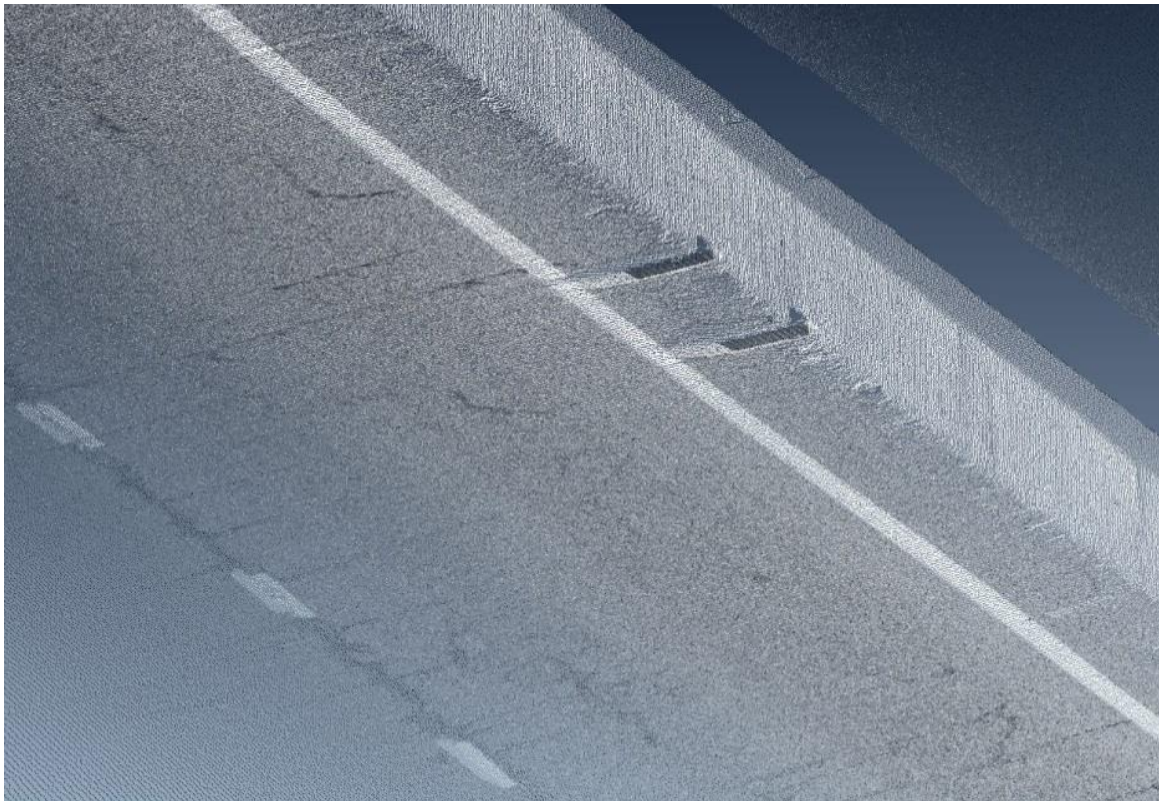
Figure 7.1. Culvert inlet in MTLs point cloud
