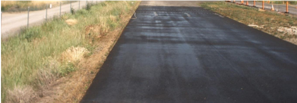
Figure C.22. Front Center Camera view
