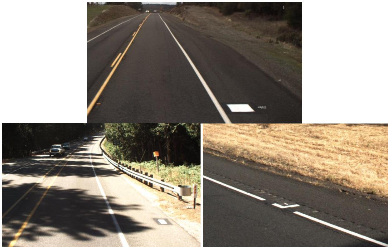
Figure 5.10. Example ground control targets located on the road shoulder
