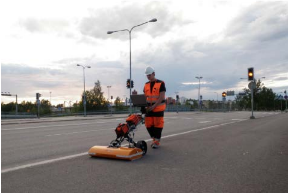
Figure 24: The deck was also measured using the new system of IDS (Ingegneria dei Sistemia Inc., Roadscanners)
