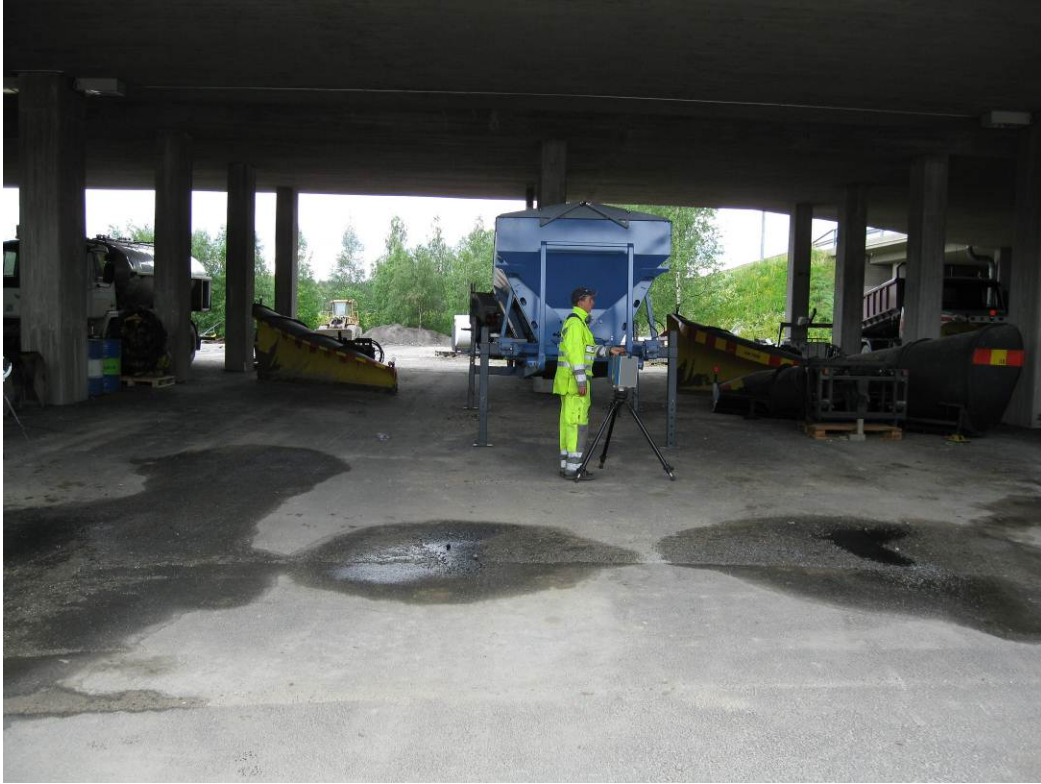
Figure 20: Measuring under the bridge deck
