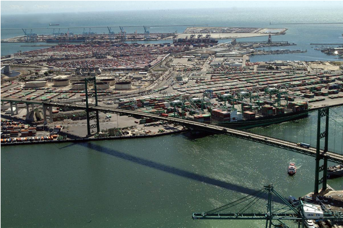
Figure 5: Vincent Thomas Bridge, Los Angeles, California
