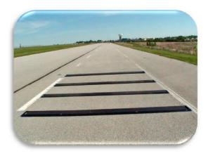
Figure 5. Portable Plastic Rumble Strips.
