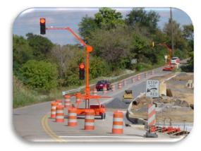
Portable traffic signals are traffic signals mounted on trailers that can be used to control the right-ofway in a work zone. Communications between the signals are provided by hard wiring, radio frequency transceiver, or by preset timing. Thus, portable traffic signals can actually replace flaggers; thereby, removing flaggers from direct exposure to approaching traffic and allowing flaggers to perform other critical work tasks.
