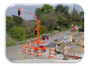
Figure 11. Portable Traffic Signal.
