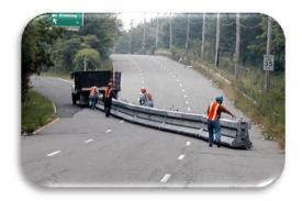
Some steel barrier designs include retractable wheels
