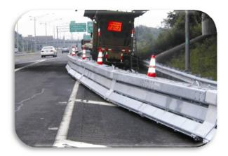
Figure 9. Example of Steel Barrier.
