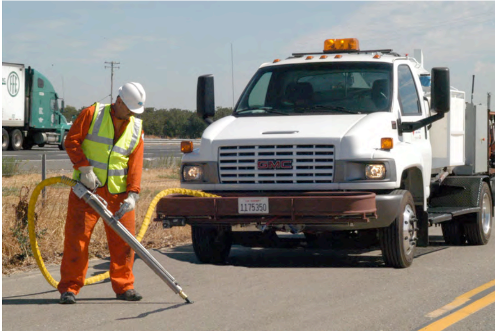
Figure 11. Sealzall In-Lane Sealing
