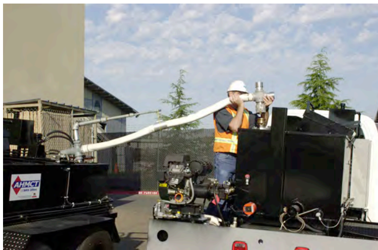
Figure 3. TTLS Sealant Transfer
