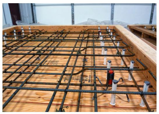
Figure 12: Close-up of reinforcement layout.
