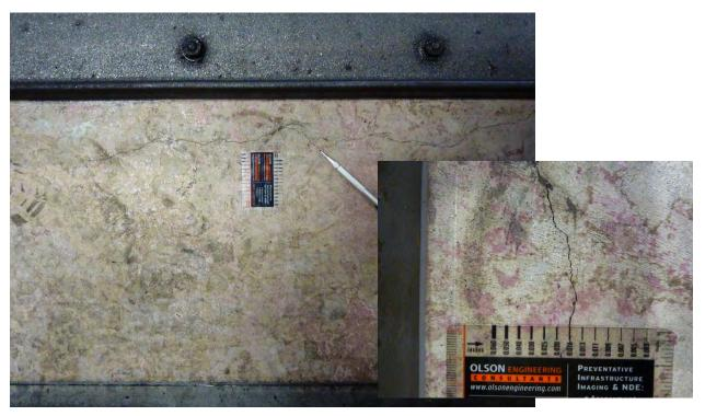
Figure 37: Longitudinal crack in top surface.
