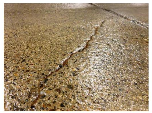
Figure 34: Close-up of methacrylate-filled crack.
