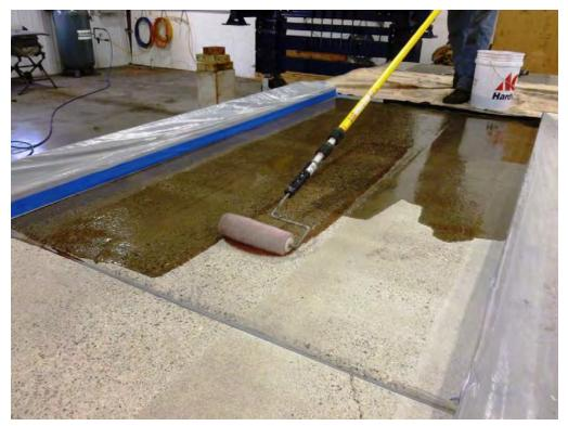
Figure 33: Application of HMWM surface treatment.
