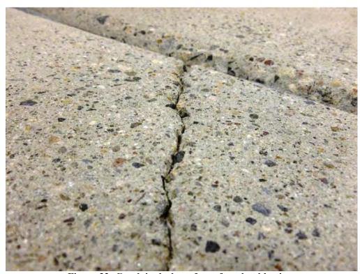
Figure 32: Crack in deck surface after shot blasting.
