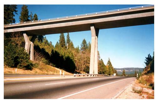
Figure 1: Concrete box girder bridge in Nevada County, CA (photo by Mark Yashinsky<sup>1</sup>)
