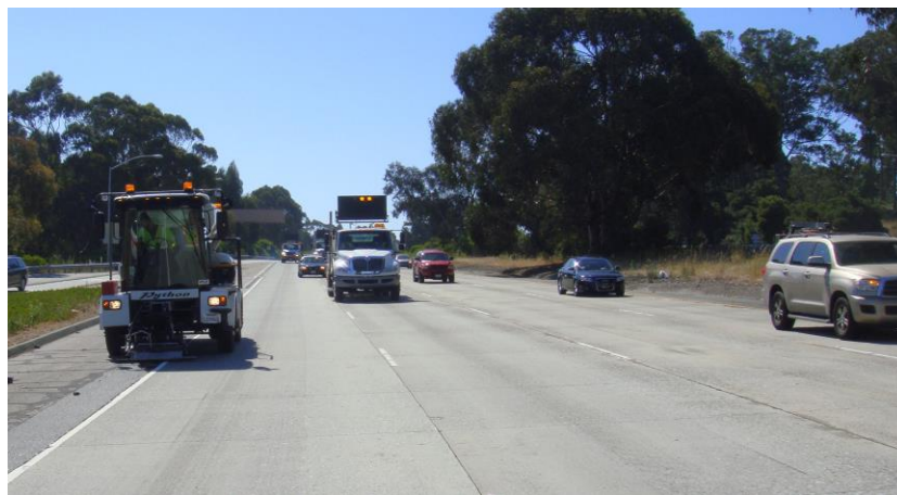
Figure 4. Caltrans Moving Closure Patching Operation
