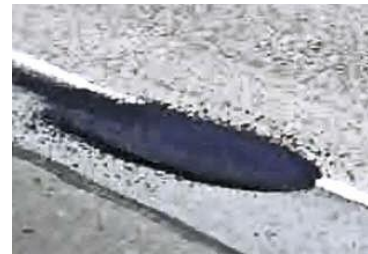
Figure 8. Hot Asphalt Patch
