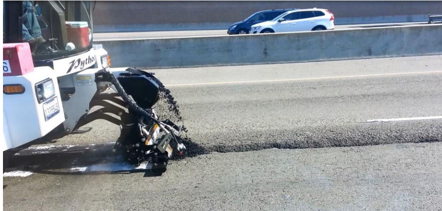
Figure 21. Linear Pavement Gap Patching
