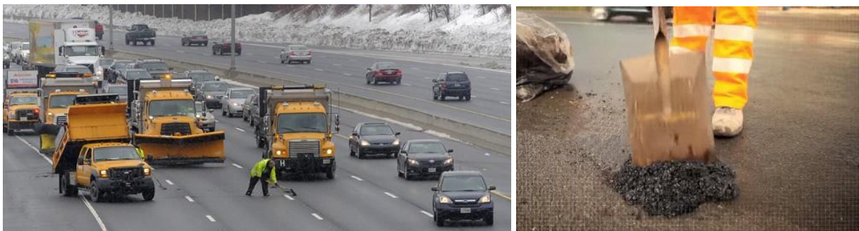
Figure 1. Manual Pothole Patching on Mainline Highway
