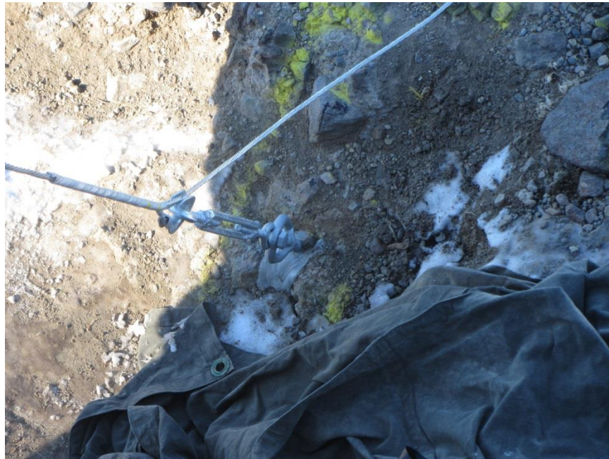
Figure 3.34: A close-up of the north tower anchor
