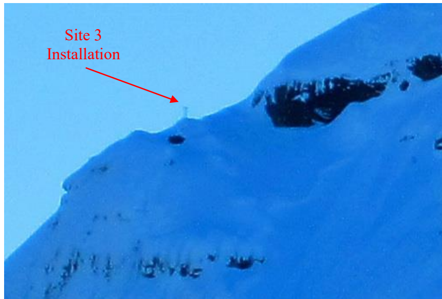
Figure E.2: Winter 2014 close-up of site installation. The tower is visible near the image center.
