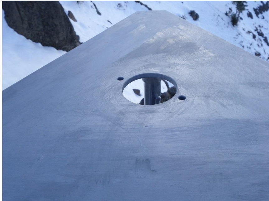
Figure 3.39: The top plate with mounting for the wind generator mast
