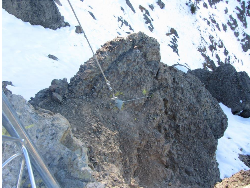
Figure 3.31: The southwest tower anchor
