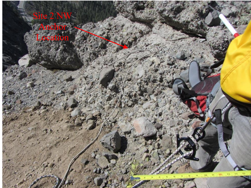
Figure 3.25: The northwest anchor location at the second site
