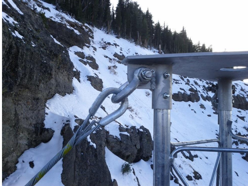
Figure 3.38: A close-up of the anchor plate and guy wire attachment
