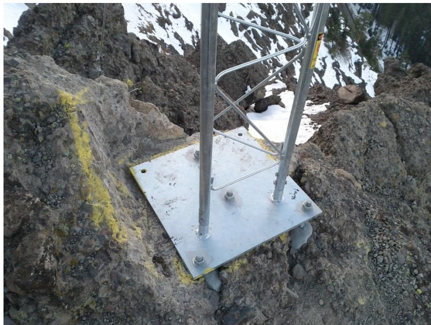
Figure 3.30: The tower base bolted to the rock conglomerate
