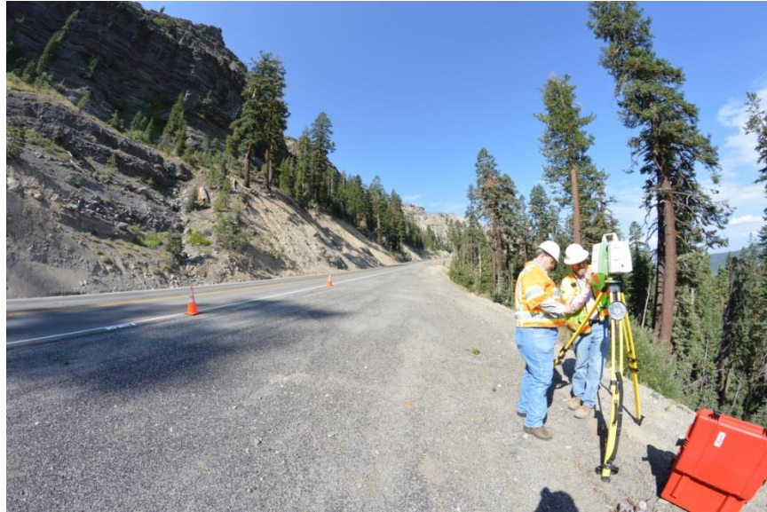
Figure 3.4: Surveying from the roadway below Carson Spur chute 4
