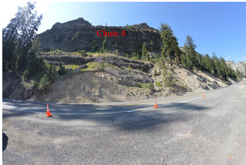
Figure 3.3: View of Carson Spur chute 4 from the roadway
