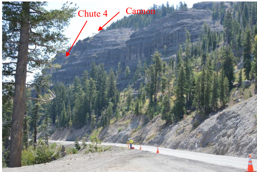
Figure 3.5: Surveying avalanche zones along Carson Spur with chute 4 in the distance and a Gazex cannon visible on the rock face
