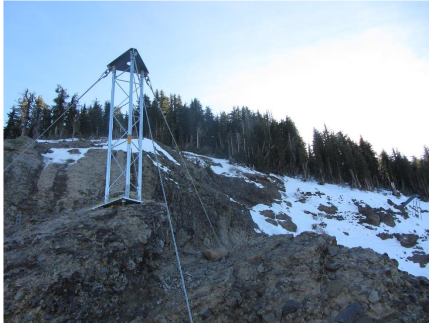
Figure 3.29: The south view of the final site's tower installation
