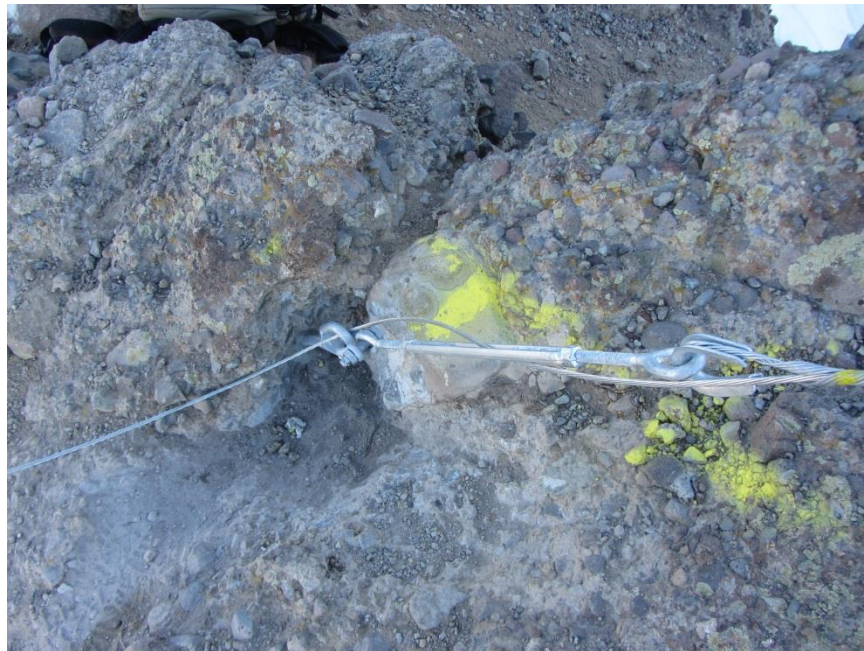
Figure 3.36: A close-up of the southeast tower anchor
