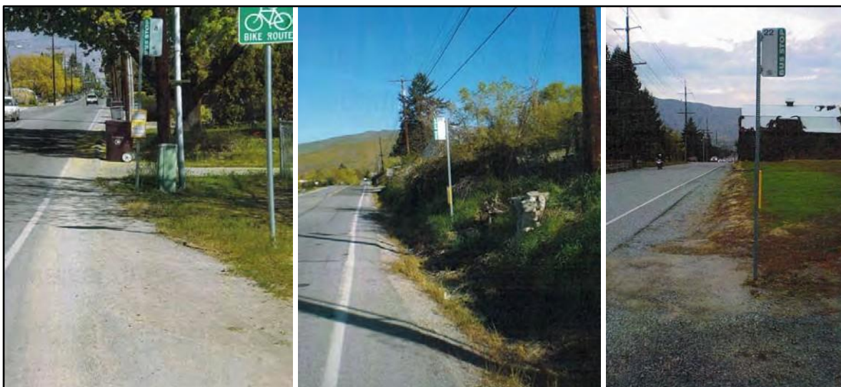
Figure 38. Rural Bus Stop Infrastructure Conditions
