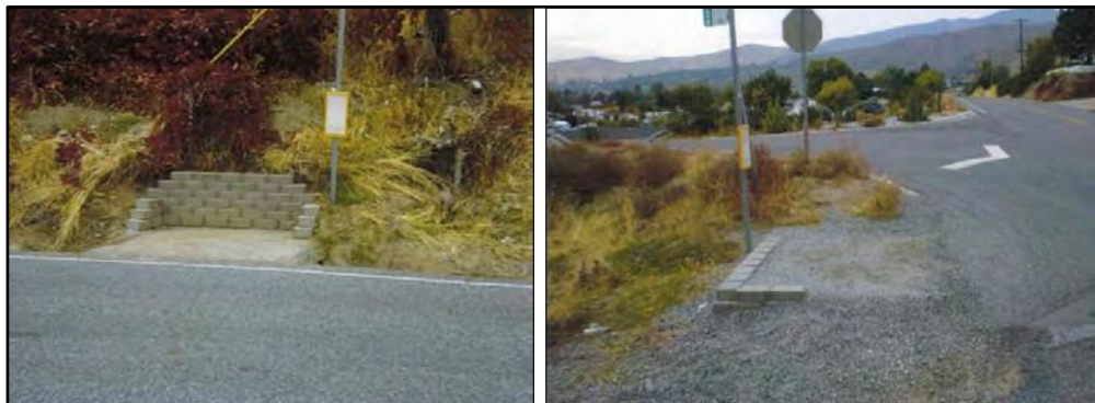
Figure 39. Rural Bus Stops Improved Using "Rhino Snot"
