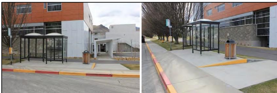
Figure 40. Wenatchee Hospital Transit Stop at Main Entrance
