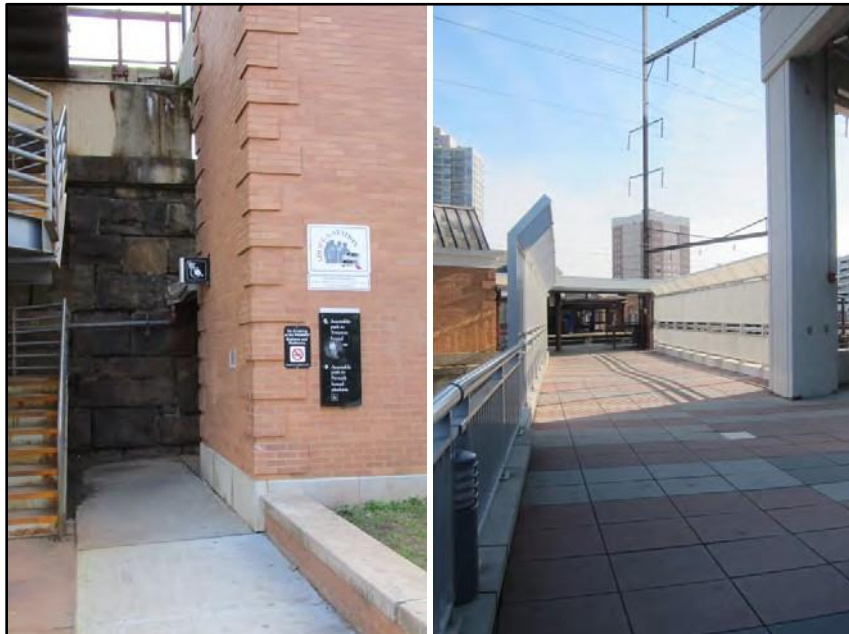
Figure 27. (Left) Outbound Elevator/Stairs; (Right) Ramp Connecting Somerset Street to Outbound Platform (Elevators are Located to the Right), New Brunswick Station, New Brunswick, NJ
