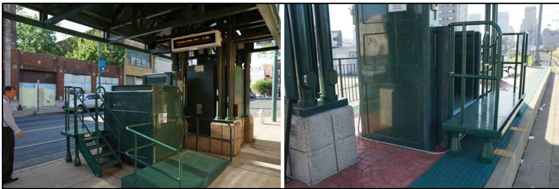
Figure 22. (Left) Trolley Station with Mechanical Lift and Variable Message Sign; (Right) Trolley Station Wheelchair Boarding Platform and Textured Ground Surface
