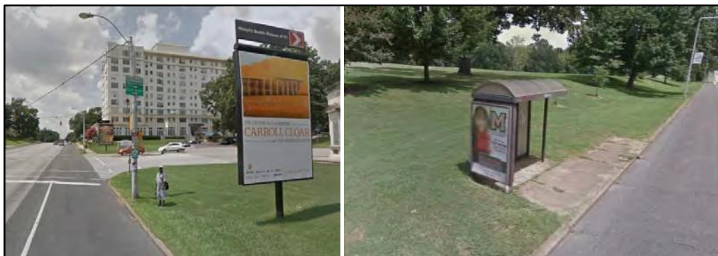
Figure 20. (Left) Discontinuous Sidewalk; (Right) Inaccessible Bus Stop for Wheelchair Users
