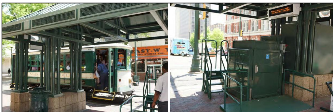
Figure 18. (Left) Downtown Trolley Station; (Right) Wheelchair Lift and Variable Message Sign at Downtown Trolley Station
