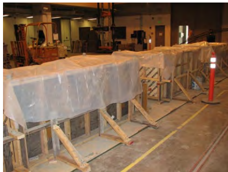
(e) Curing concrete
