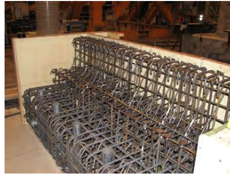
(b) Specimen S1 reinforcement
