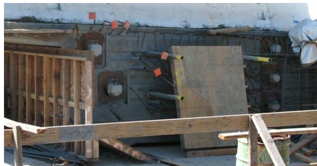
(b) Post-tensioned anchorage and connection steel
