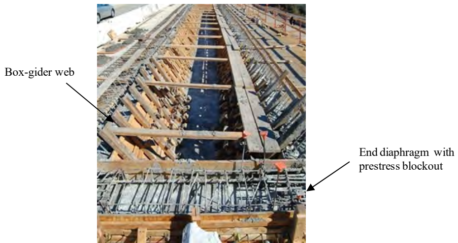
(a) Construction process
