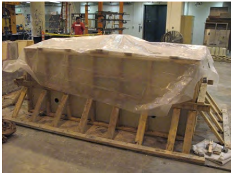
(e) Curing concrete
