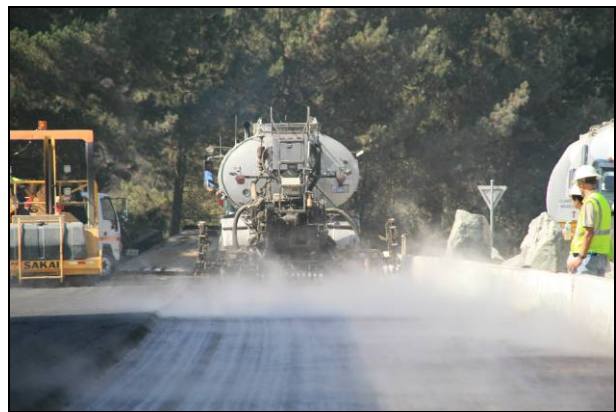
Figure 2.42: Tack coat application (Sasobit).
