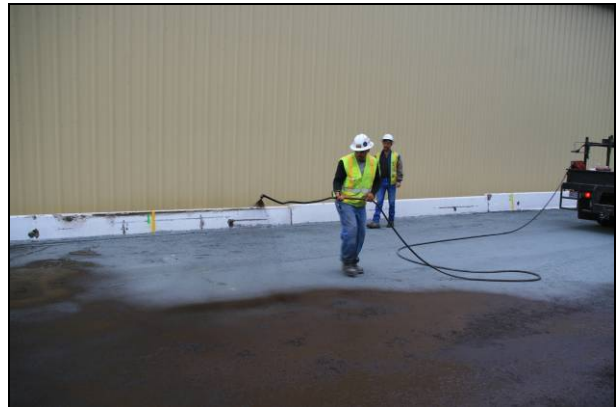
Figure 2.27: Prime application.
