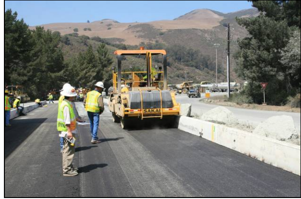
Figure 2.36: Evotherm: Surface after final rolling.
