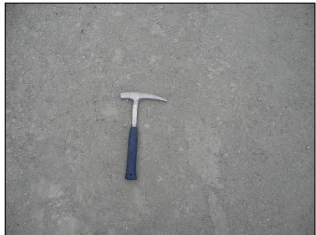
Figure 2.11: Completed base-course showing tightly bound surface.
