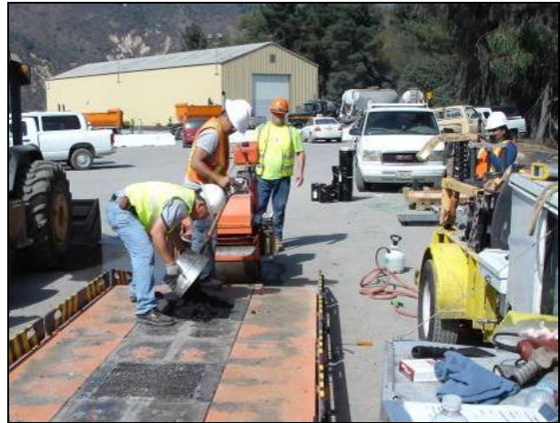
Placing sample in mold
