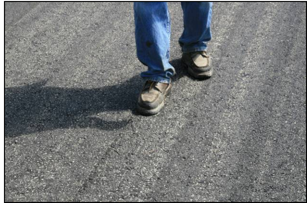
Figure 2.40: Sasobit: Shearing during final rolling.
