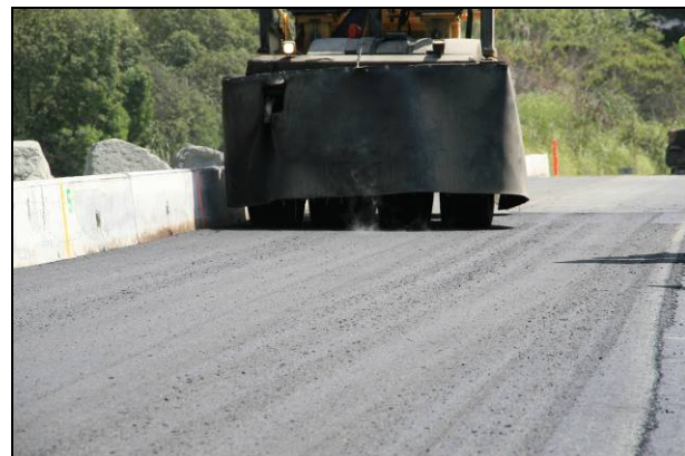
Figure 2.38: Sasobit: Pick up during rubber-tire rolling.
