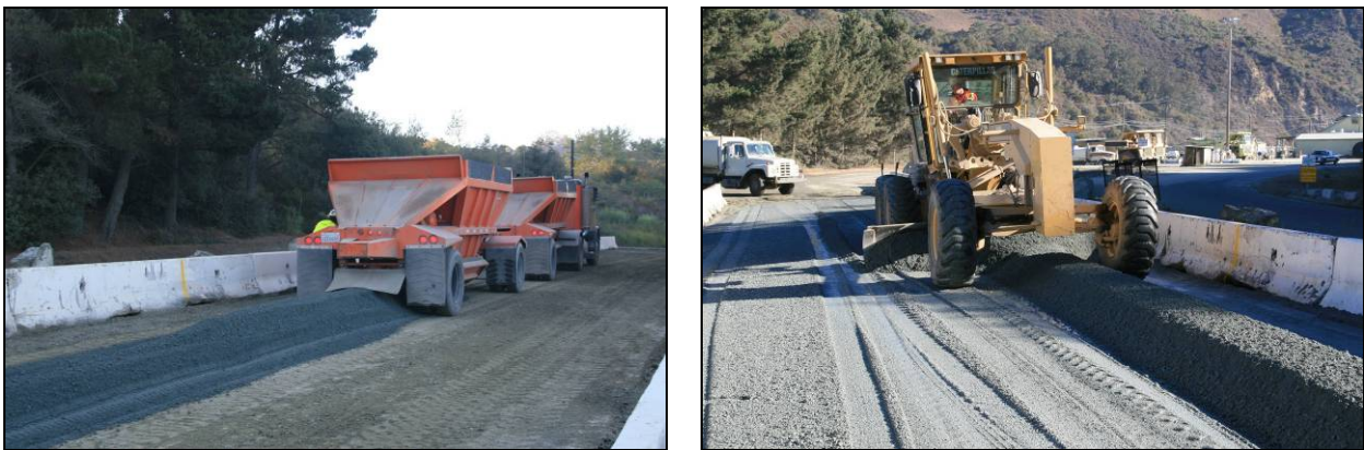
Figure 2.8: Base-course construction.
