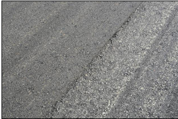
Figure 2.39: Sasobit: Surface after final rolling.
