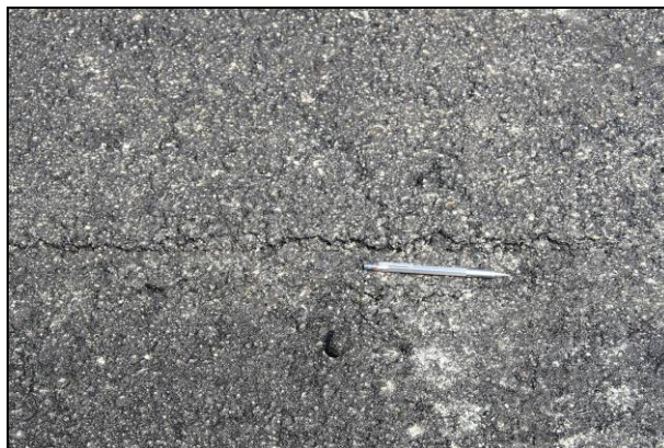
Figure 2.37: Sasobit: Shearing during breakdown rolling.
