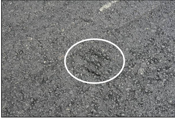
Figure 2.35: Evotherm: Shear after rubber-tired roller.
