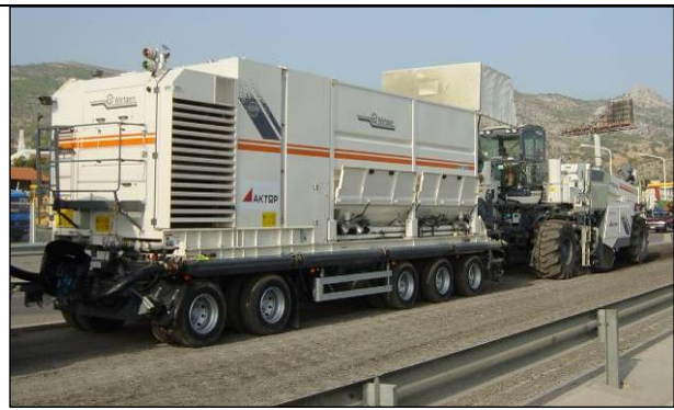
(b) Rotary mixer/recycler coupled to slurry applicator
