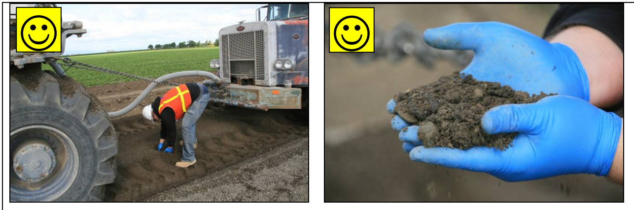
Figure 7.6: Checking material consistency and color.
