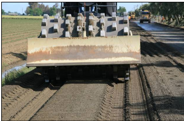
Figure 7.9: First padfoot roller pass.
