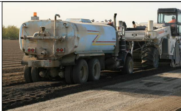
(a) Rotary mixer/recycler coupled to water tanker
