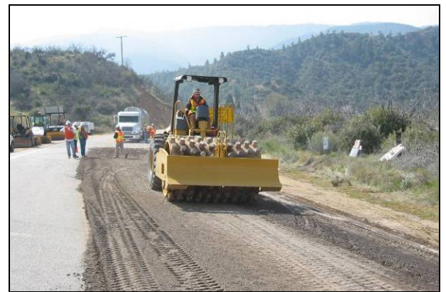
Figure 7.12: Padfoot impressions after multiple passes.
