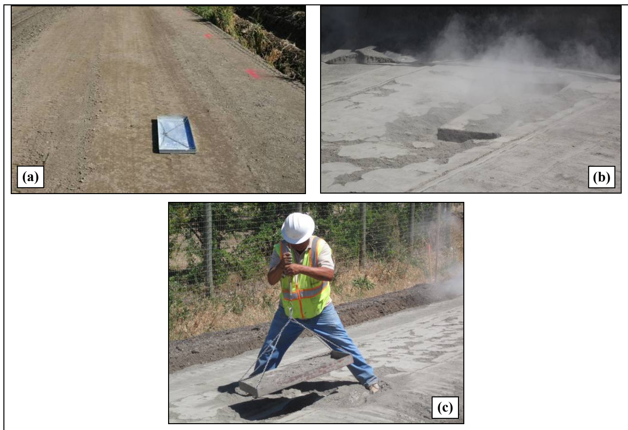
Figure 7.4: Monitoring stabilizer application rate.
