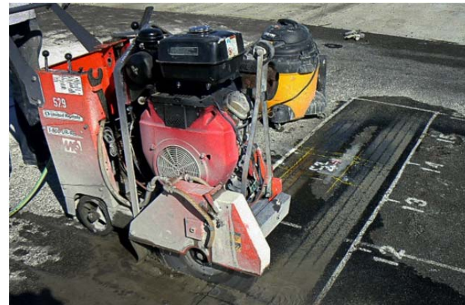
(i) Removal of scanned blocks for post-test scanning
