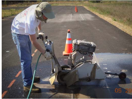
(b) Sawing of blocks
