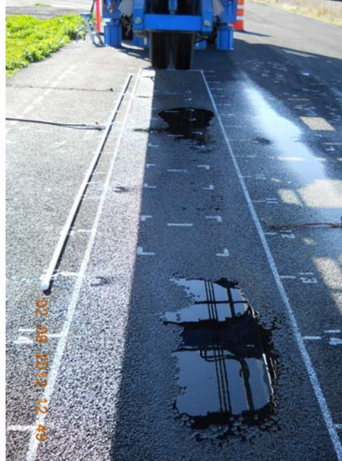
(c) Water sprayed onto pavement with perforated PVC pipe
