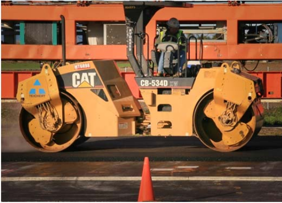
(a) Construction of OGFC
