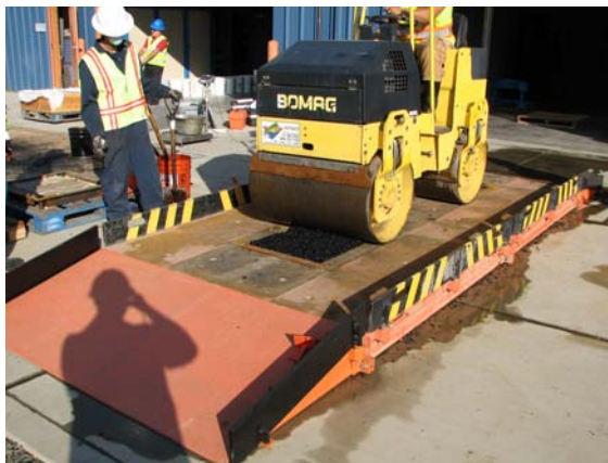
(a) Compaction using rolling wheel
