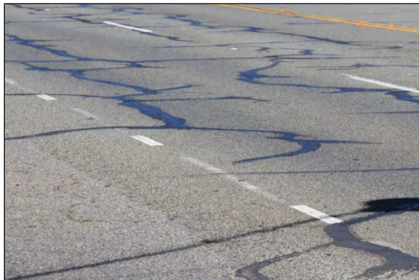
Figure 8.1: Auburn Evotherm, July 2010, one month prior to paving.
