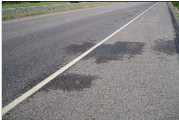
Figure 3.16: Morro Bay Sasobit, June 2013 (73 months), showing effective drainage.
