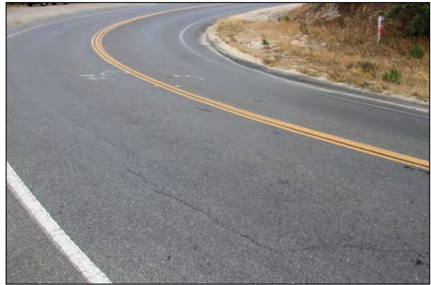
Figure 4.3: Point Arena Evotherm, November 2010, showing longitudinal cracks.
