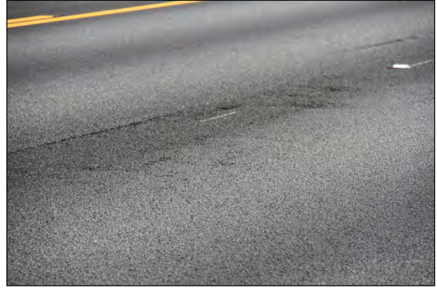
Figure 8.2: Auburn Evotherm, August 2010 (0 months). Note segregation and open joint.
