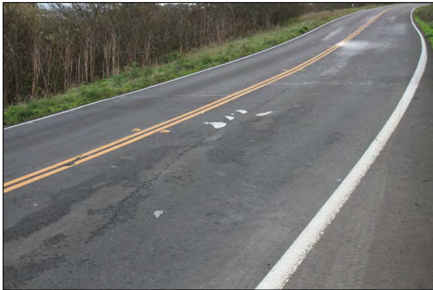
Figure 4.3: Point Arena Evotherm, November 2010, showing longitudinal cracks.
