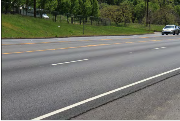
Figure 8.2: Auburn Evotherm, August 2010 (0 months). Note segregation and open joint.
