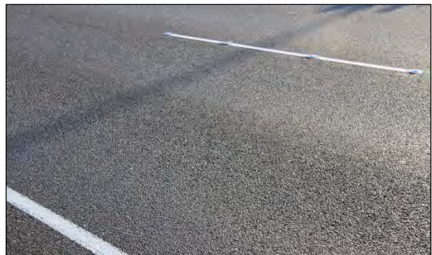
Figure 5.4: Orland Evotherm, June 2011 (24 months). Note ruts in wheelpath.
