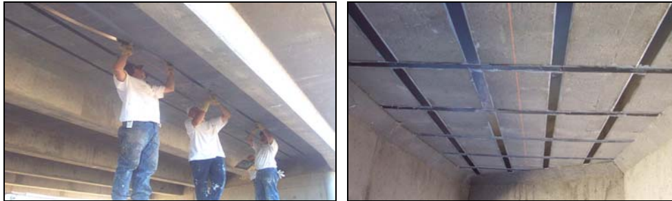
Figure 6.11. Pultruded Strip Construction
