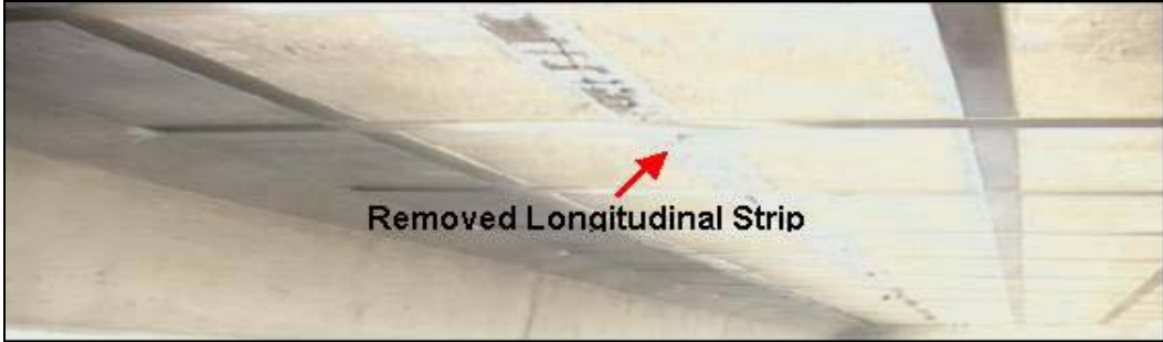
Figure 10.2. Removal of Longitudinal CFRP Strip in Location S8B1
