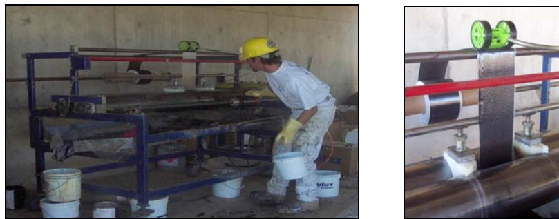
Figure 6.9. Impregnator for Wet Lay-up CFRP
