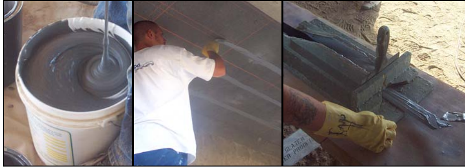
Figure 6.10. Mixing and Application of Adhesive
