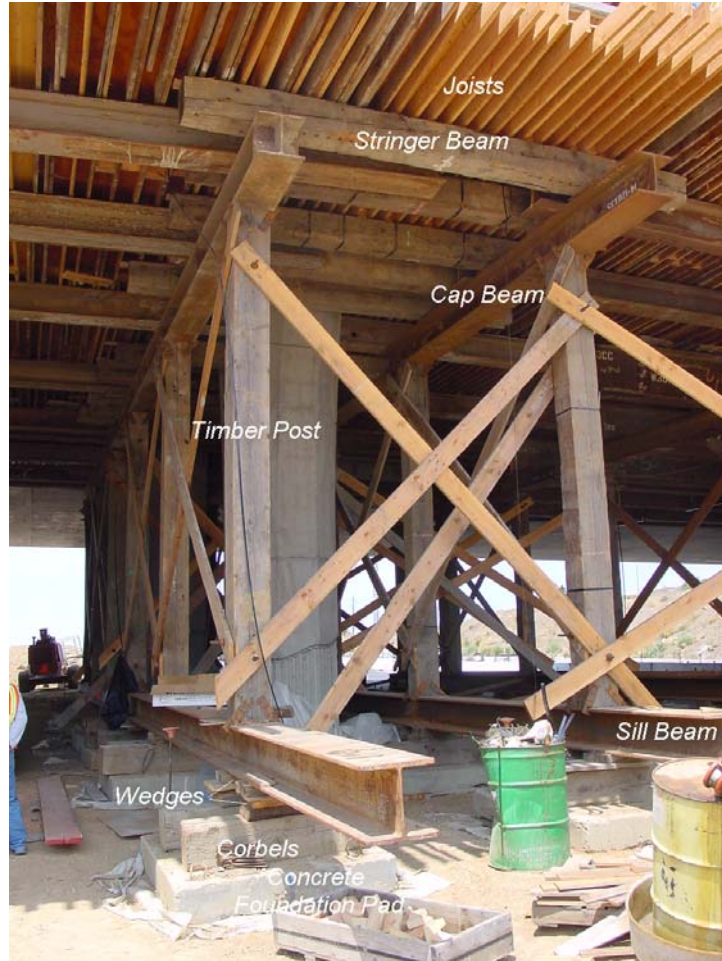
FIGURE 1-2 Bridge Falsework for Railroad Avenue Overcrossing at Pittsburg, California
