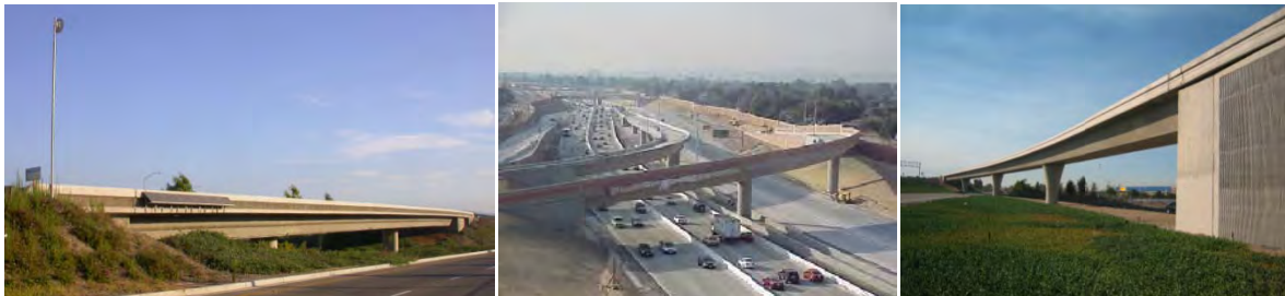
Figure 1. Three Instrumented Bridges.
