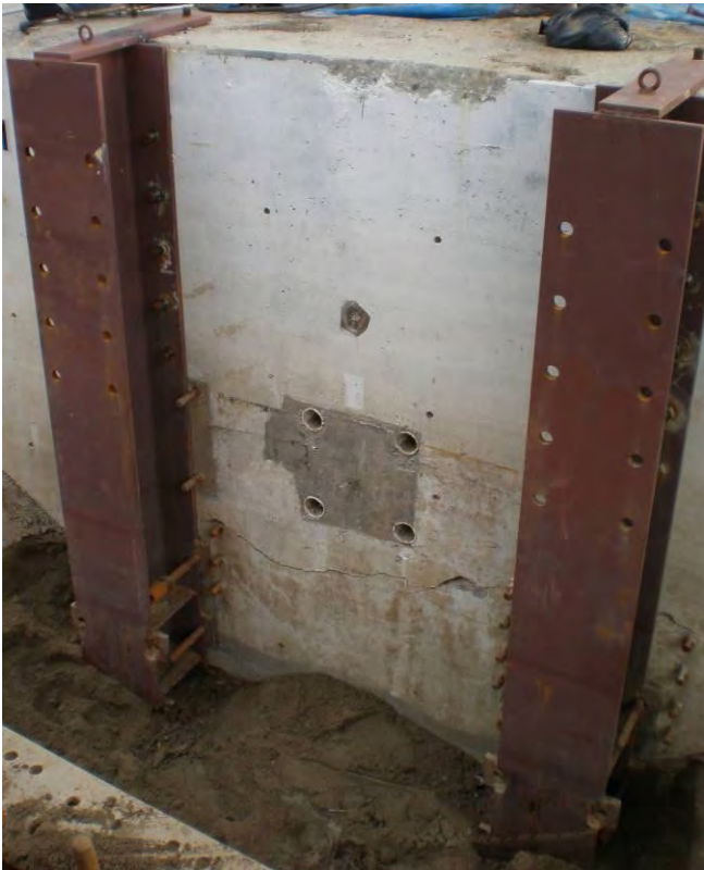
Figure 3.9 W14X120 Sections to Strengthen Damaged Backwall
