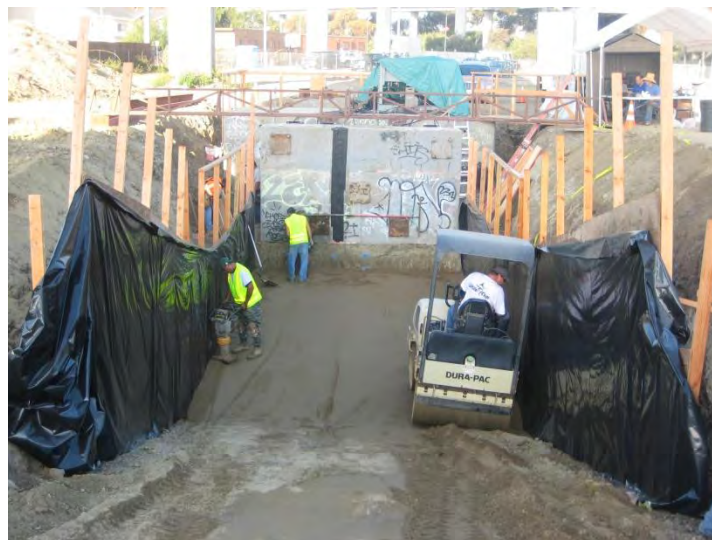
Figure 4.4a Vibratory Drum Roller Compacting a Lift for T8.0-1
