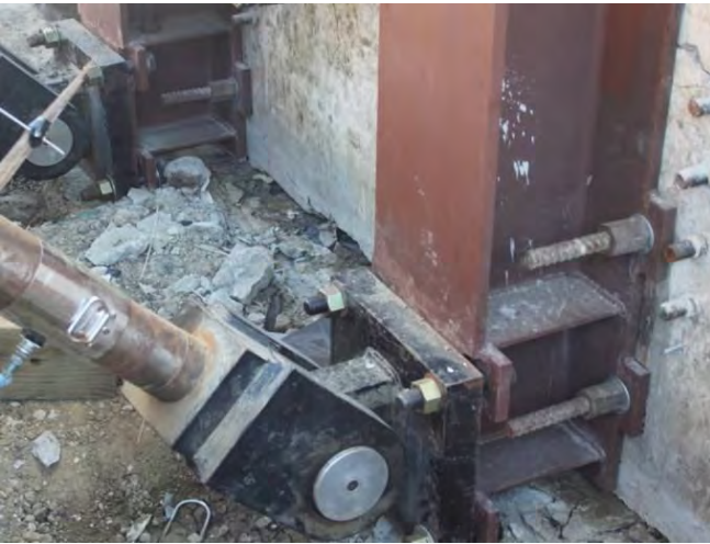
Figure 3.10 Diagonal Actuator Attached to W14X120 Steel Sections
