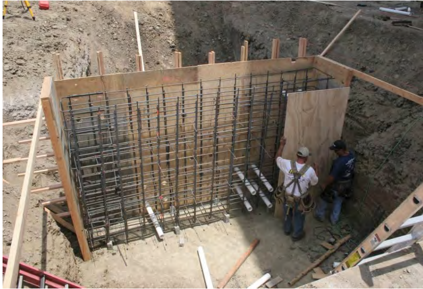
Figure 4.2 Abutment Wall Reinforcement Cage
