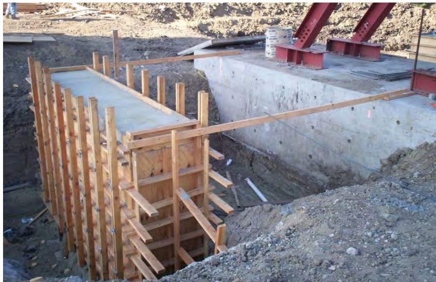
Figure 4.3 Formwork and Concrete Curing
