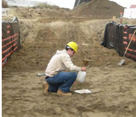
Figure 4.9 Sand Cone Testing between Lifts
