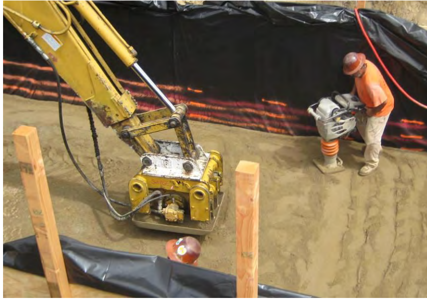
Figure 4.5b Hydraulic Vibrator and Manual “Whacker” Compacting a Lift (T8.0-2)
