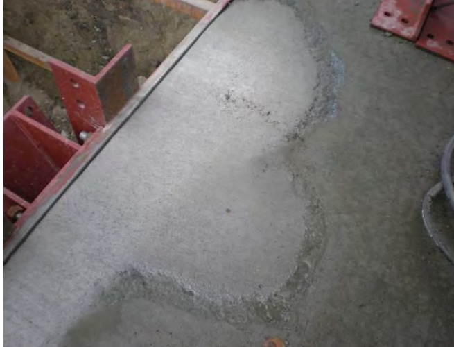
Figure 3.12 Repaired Edge of Concrete Reaction Block
