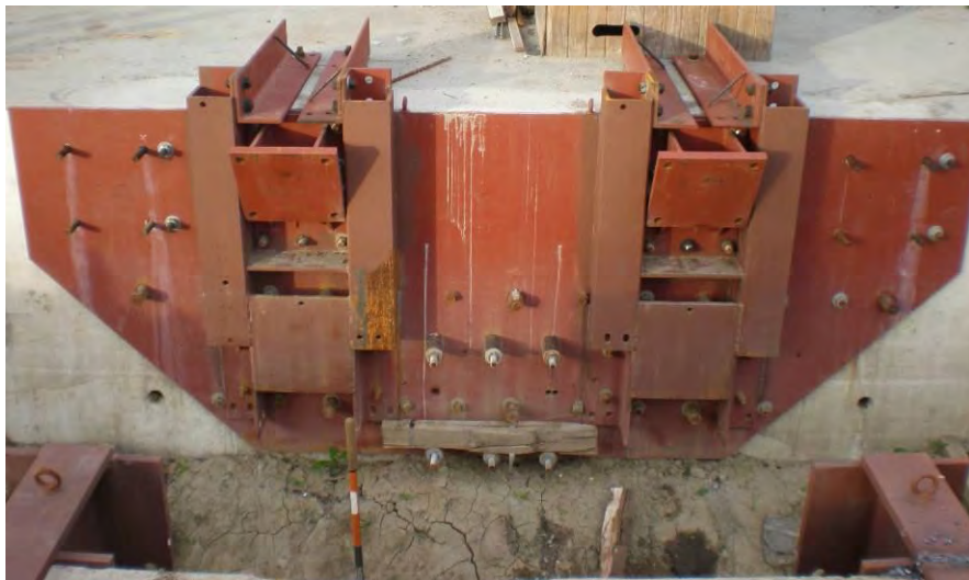
Figure 3.11 Steel Plate and Angle Assembly to Strengthen Reaction Block
