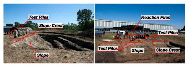
Figure 4-8. Overall view of the completed slope excavation (Stage 1)
