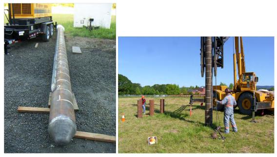
Figure 4-11. Installation of Baseline Pile (I-1)
