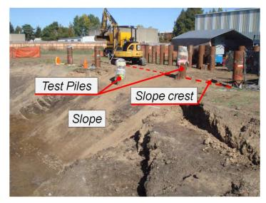
Figure 4-10. Overall View of the completed slope excavation in Stage 2 of Series-I
