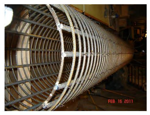
Figure 4.5.1. Reinforcement Cage during Construction
