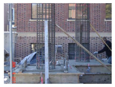
Figure 4.5.4. Cast Footing and Column Reinforcement Cage
