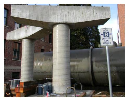
Figure 4.5.7. Completed Single-Column Bents
