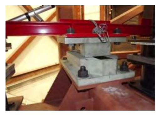
Figure 4.4.4. Assembled Shear Key Installed Between Bottom Chord of Cross-Frame and Abutment Seat
