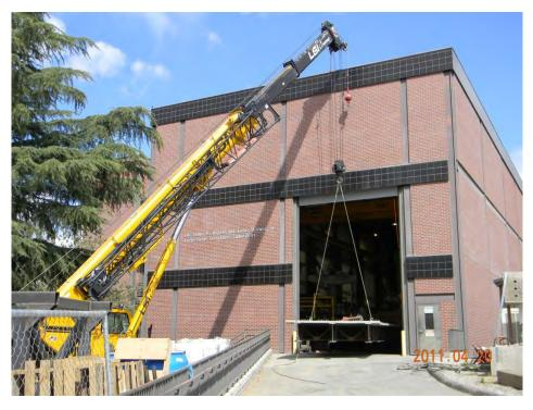
Figure 4.5.11. Moving Superstructure Segment into the Laboratory
