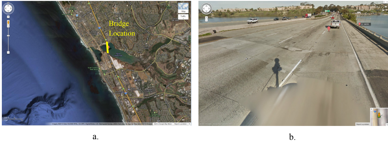
Figure 25. a) Location of the Agua Hedionda Lagoon Bridge, b) close-up view of the bridge (Source: Google maps).
